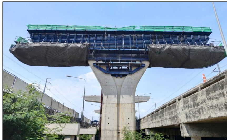
Install Steel Crossbeam Pier Type Y-5 MLP06-07C
