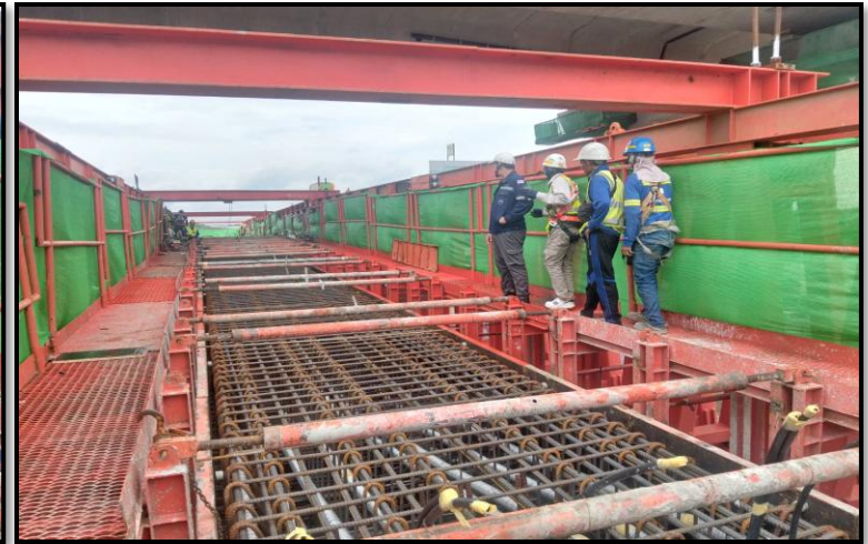
MLP01-08 Final Inspection Lower Crossbeam Type PTT-1
