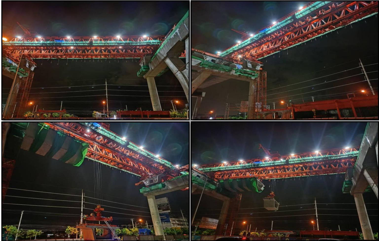
MLP03-27 to MLP03-28 Erection segment (LG4)
