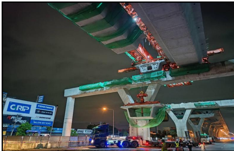
MLP01-27 to MLP01-28 Erection Segment (LG2)
