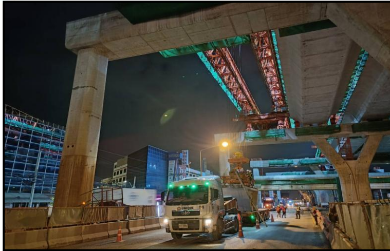
MLP01-25 to MLP01-26 Erection Segment (LG1)
