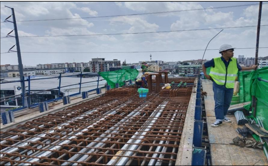
Install Steel Crossbeam Pier Type Y-5 MLP06-07C
