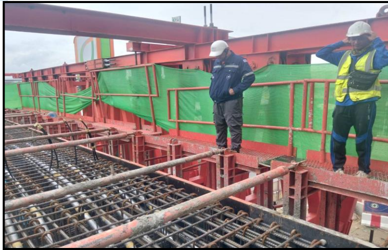
MLP01-08 Final Inspection Lower Crossbeam Type PTT-1
