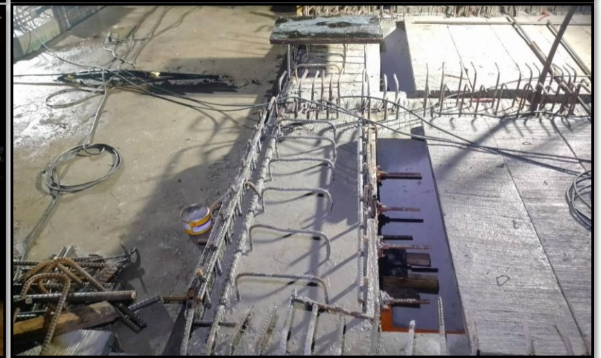
Pouring Concrete Girder Diaphragm ROF2-07 to ROF2-08
