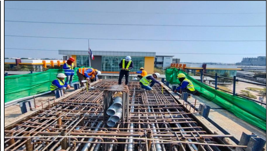
Install Steel Crossbeam Pier Type Y-5 MLP06-09C
