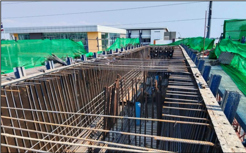
Install Steel Crossbeam Pier Type Y-5 MLP06-08C
