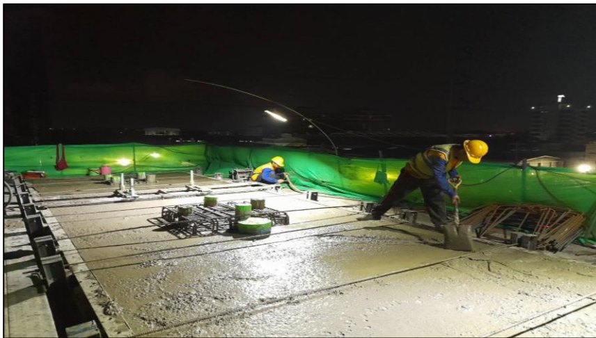
Pouring Concrete Crossbeam Pier Type Y-1 MLP06-06C
