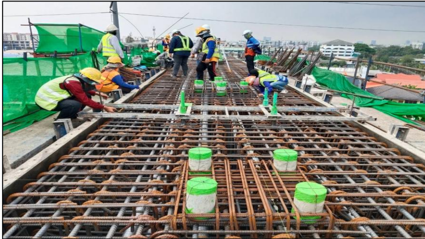
Install Steel Crossbeam Pier Type Y-1 MLP06-06C
