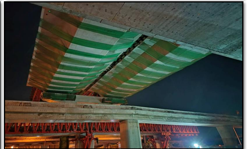
MLP01-03 to MLP01-05 Erection segment (LG1, 2)
