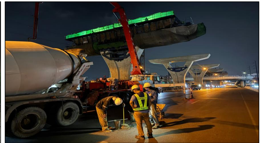
Pouring Concrete Crossbeam Pier Type Y-1 MLP06-06C
