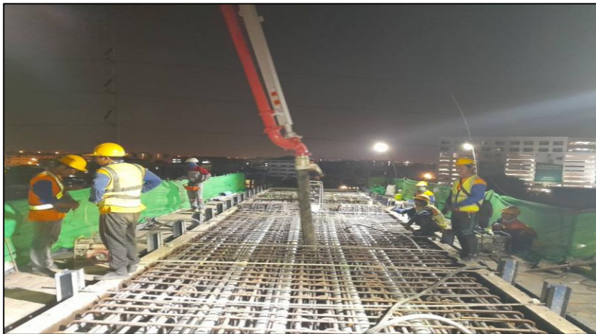
Pouring Concrete Crossbeam Pier Type Y-5 MLP06-09C Step 1
