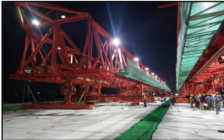
MLP04-09 to MLP04-10 - Launching gantry back (LG3,4)
