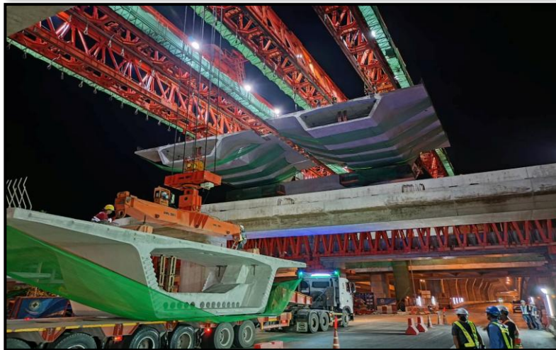
MLP01-03 to MLP01-05 Erection segment (LG1, 2)
