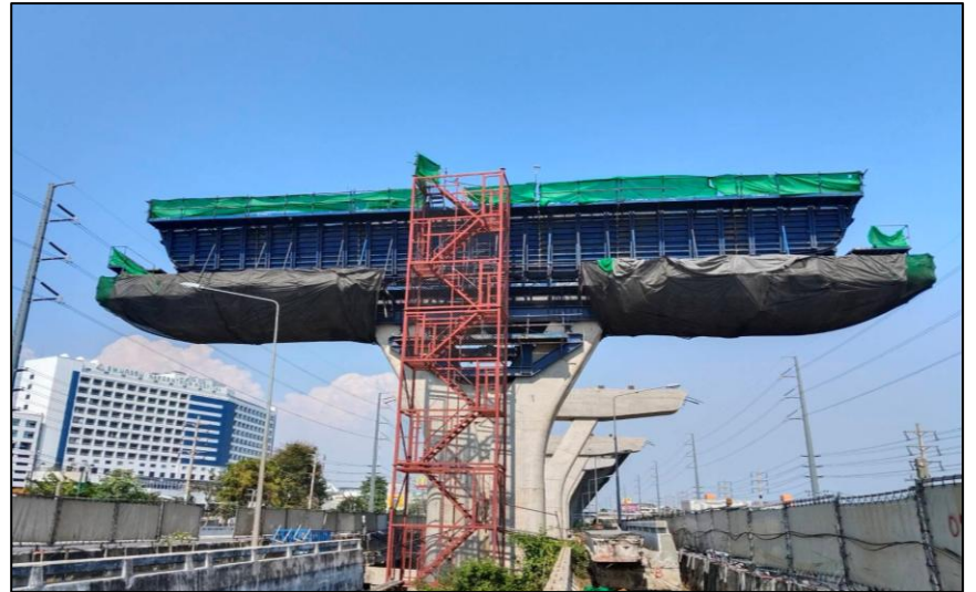
Install Steel Crossbeam Pier Type Y-5 MLP06-08C
