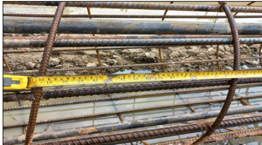
Install Rebar Bored Pile Dia 1.00 m. BP-3L/1
