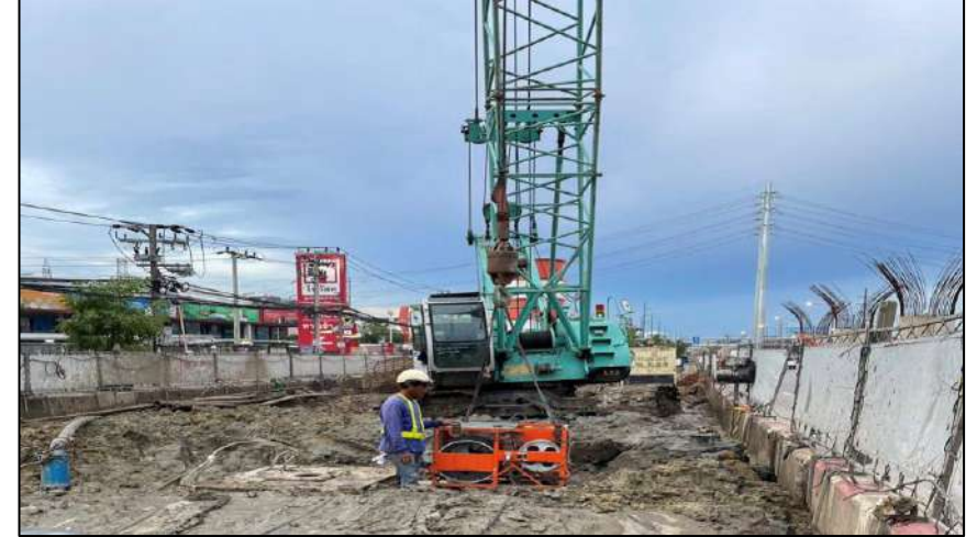
Drilling Monitor Bored Pile Test BP-6L/1
