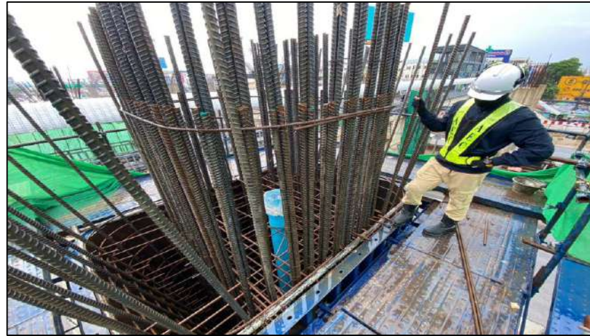
Install Steel Column Pier Type PTT-1 Step 1 MLP04-19R
