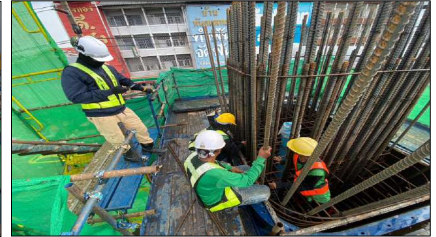
Install Steel Column Pier Type PTT-1 Step 1 MLP04-19R
