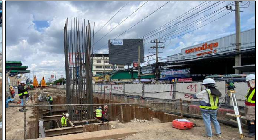
Install Steel Footing 2F3.00x1.00B MLP04-21R
