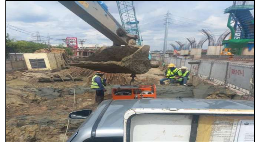
Drilling Monitor Bored Pile Test BP-1L/1
