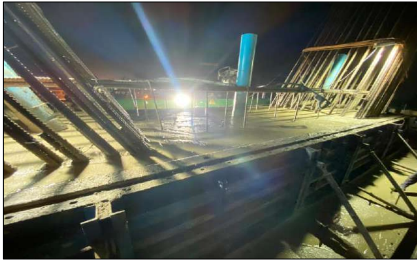
Pouring Concrete Column Pier Type YT-1 Step 3 MLP04-22C
