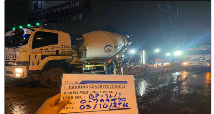
Pouring Concrete Bored Pile Dia 1.00 m. BP-1L/1
