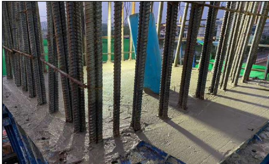
Pouring Concrete Column Pier Type Y-1 Step Y MLP04-30C
