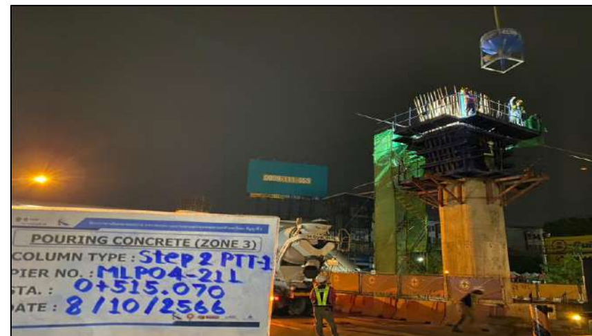
Pouring Concrete Column Pier Type PTT-1 Step 2 MLP04-21L
