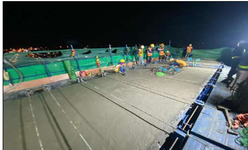
Pouring Concrete Cross Beam Pier Type Y-1 MLP04-25C
