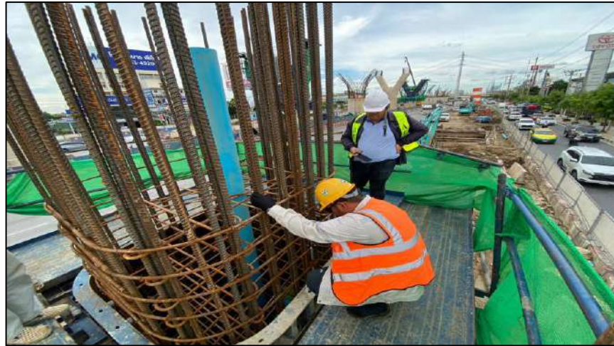
Install Steel Column Pier Type P-1 Step 1 RON2-03
