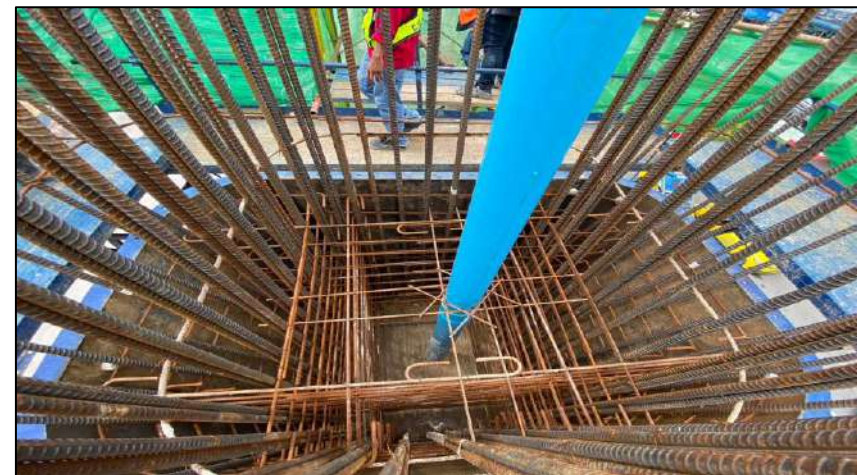
Install Steel Column Pier Type PTT-1 Step 2 MLP04-21L
