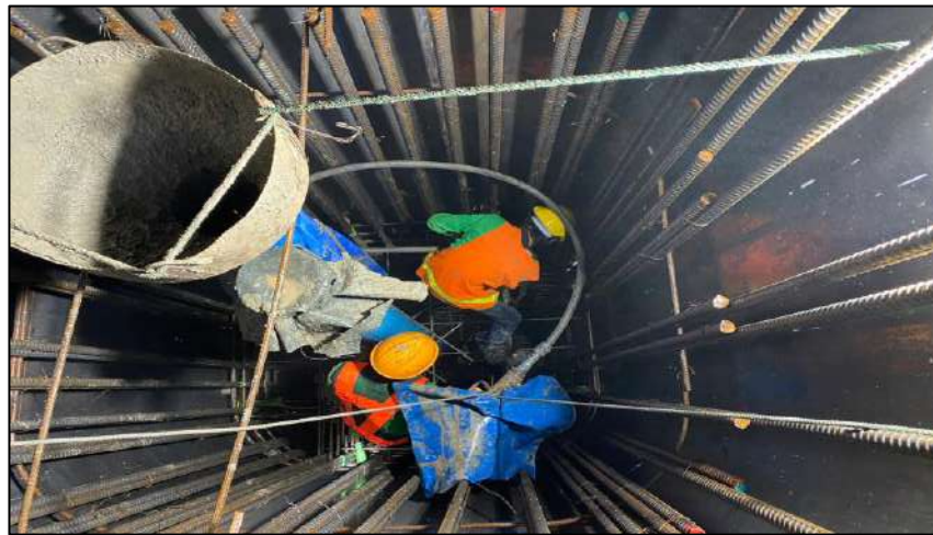
Pouring Concrete Column Pier Type PTT-1 Step 1 MLP04-20L
