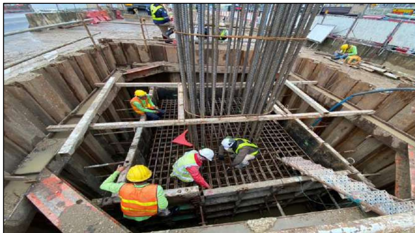
Install Steel Footing 2F3.00x1.00 MLP04-15L
