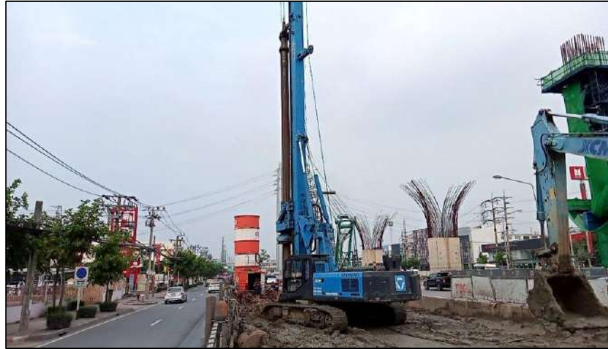
Drilling Bored Pile Dia 1.00 m. BP-6L/2
