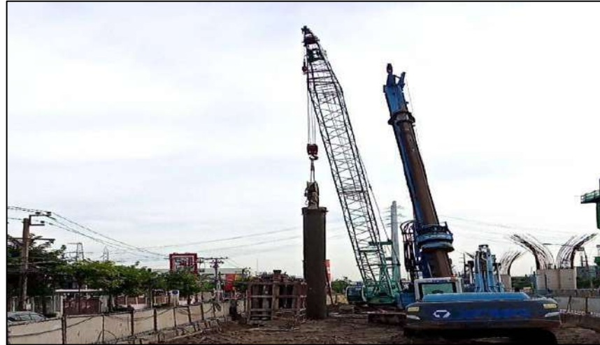
Casing Pipe at Bored Pile Dia 1.00 m. BP-4L/2
