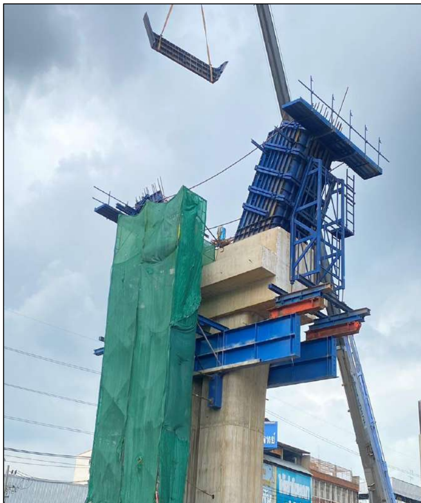
Install Steel Column Pier Type YT-1 Step Y MLP04-22C
