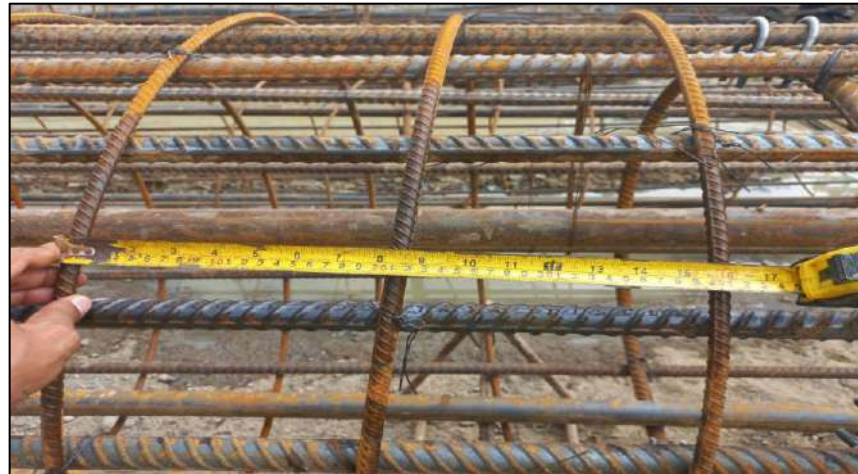
Install Rebar Bored Pile Dia 1.00 m. BP-5L/2
