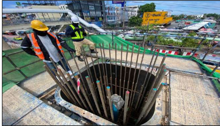
Install Steel Column Pier Type PTT-1 Step 1 MLP04-20L
