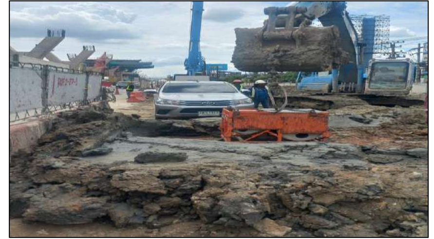
Drilling Monitor Bored Pile Test BP-2L/1
