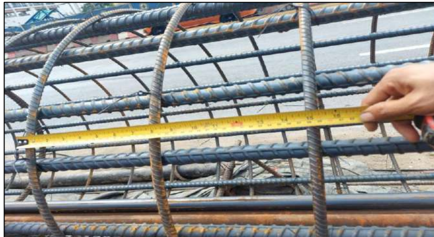
Install Rebar Bored Pile Dia 1.00 m. BP-6L/1
