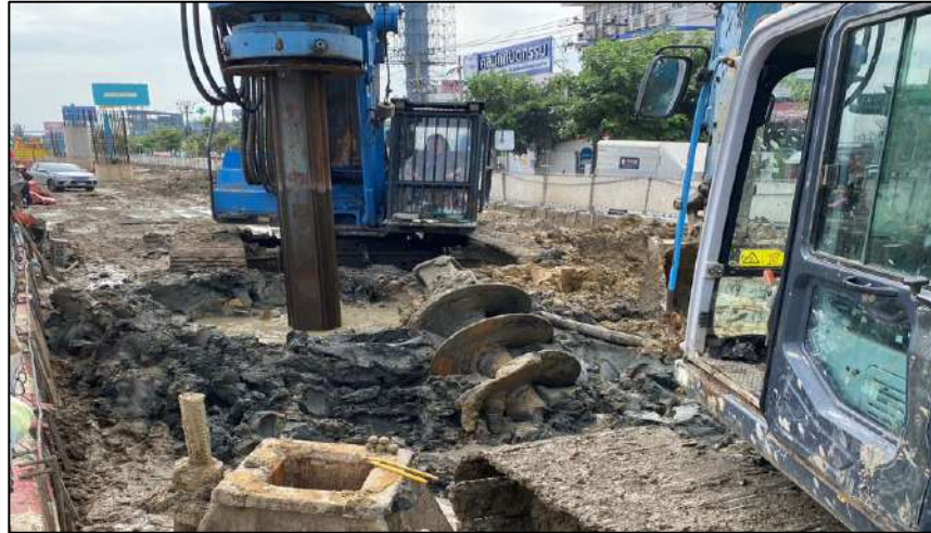
Drilling Bored Pile Dia 1.00 m. BP-2L/1
