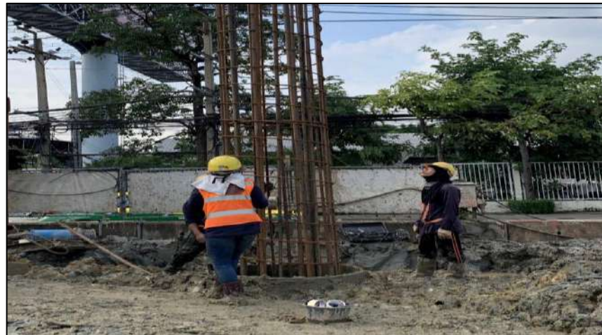
Install Rebar Bored Pile Dia 1.00 m. BP-4L/2
