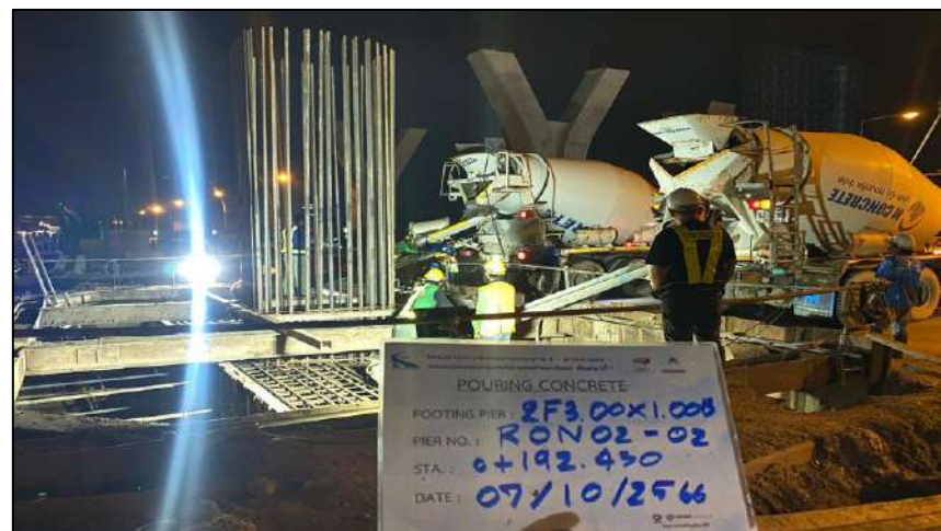
Pouring Concrete Footing 2F3.00x1.00B RON2-02
