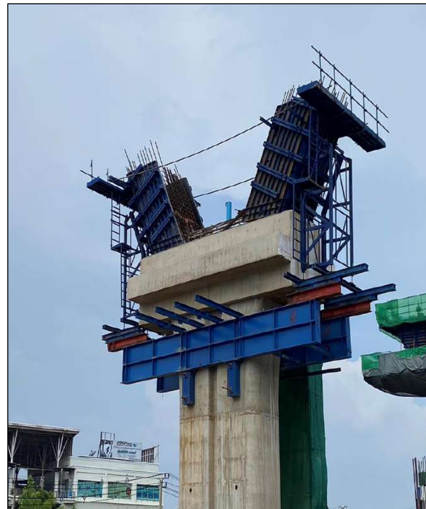
Install Steel Column Pier Type YT-1 Step Y MLP04-22C
