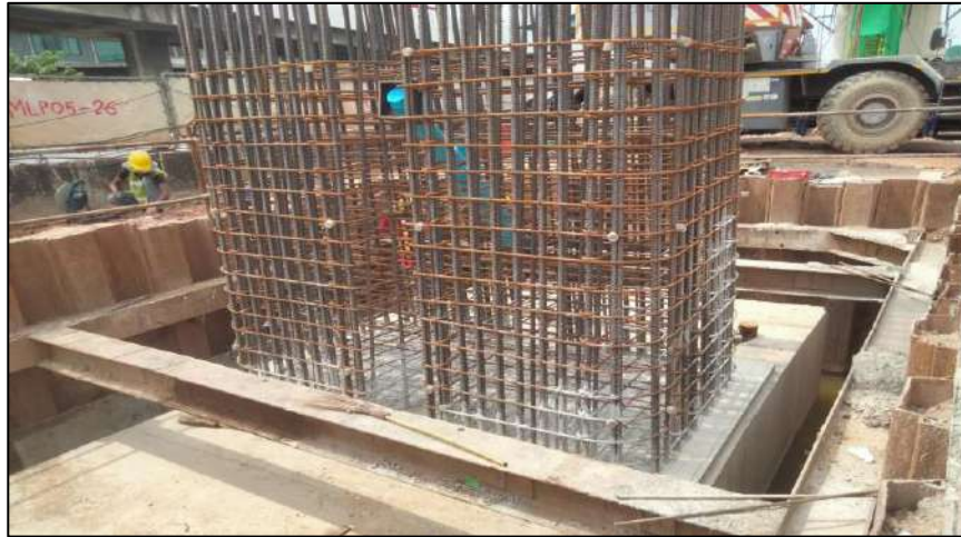
Install Steel Column Pier Type Y-3 Step 1 MLP05-26C
