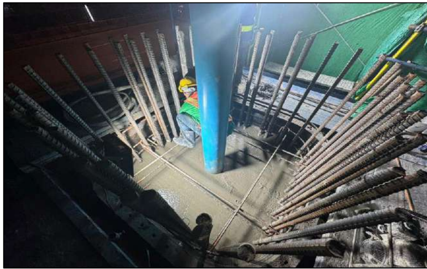
Pouring Concrete Column Pier Type P-1 Step 1 RON2-02
