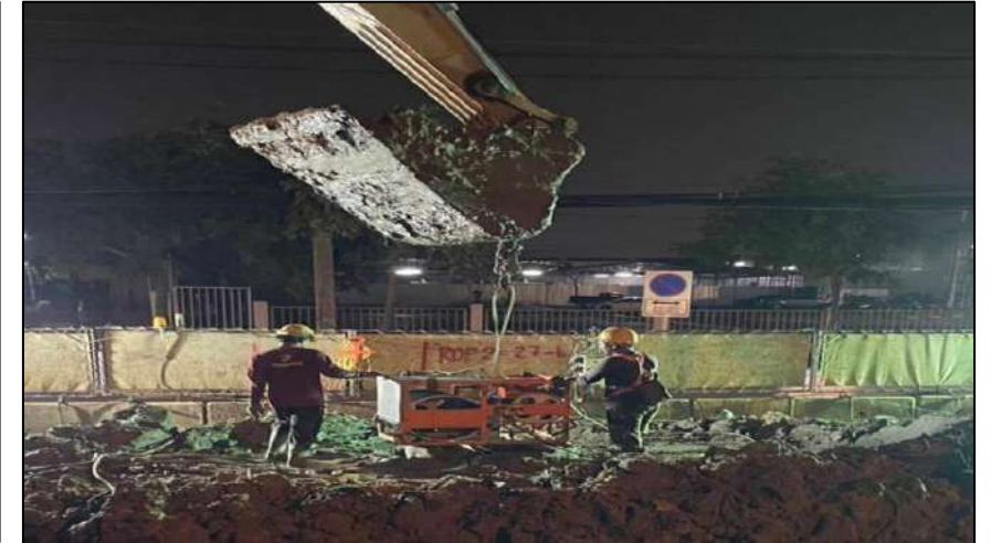
Drilling Monitor Bored Pile Test BP-6L/2
