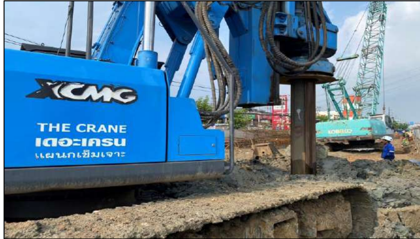
Drilling Bored Pile Dia 1.00 m. BP-6L/1
