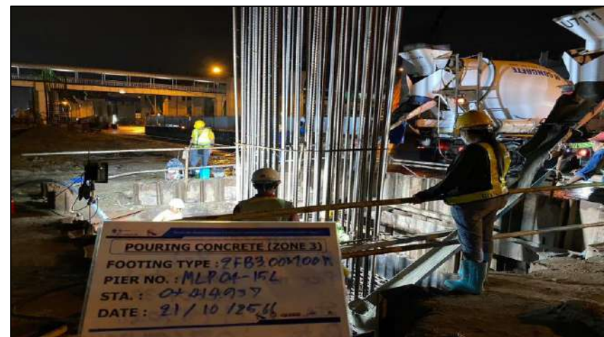
Pouring Concrete Footing 2F3.00x1.00 MLP04-15L
