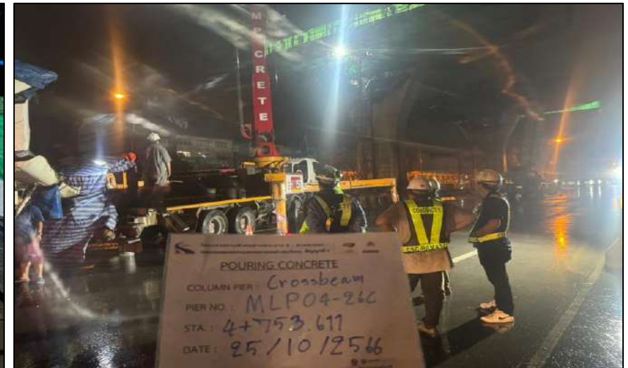
Pouring Concrete Cross Beam Pier Type Y-1 MLP04-26C
