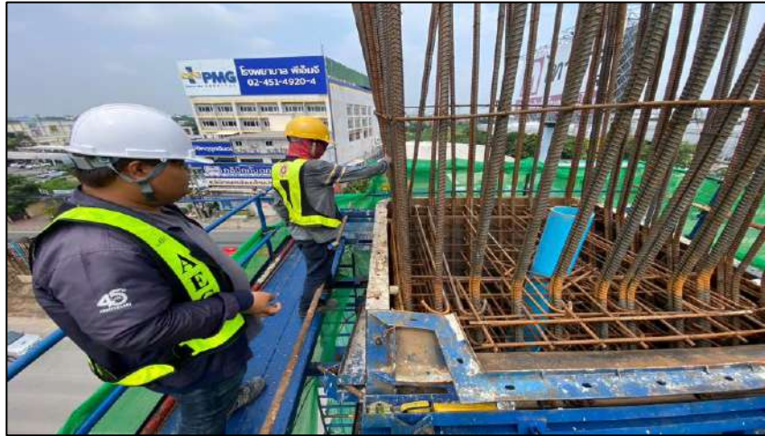
Install Steel Column Pier Type Y-1 Step Y MLP04-31C
