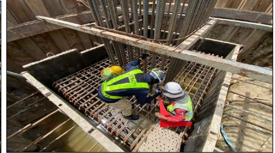
Install Steel Footing 2F3.00x1.00 MLP04-17L
