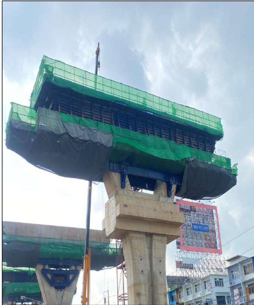
Install Steel Cross Beam Pier Type Y-1 MLP04-24C
