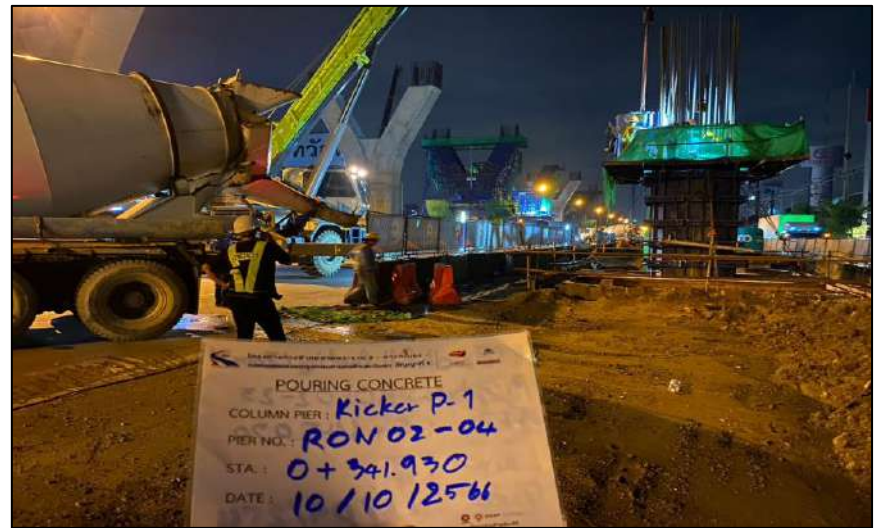
Pouring Concrete Column Pier Type P-1 Step 1 RON2-04
