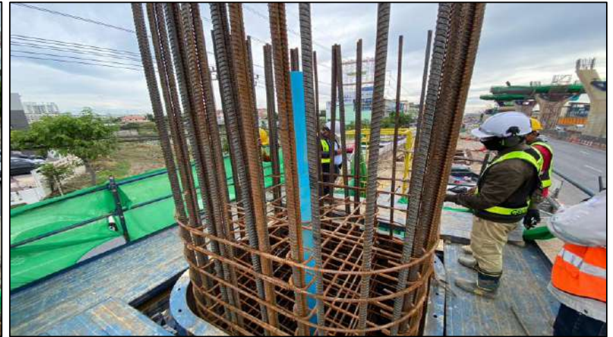
Install Steel Column Pier Type P-1 Step 1 RON2-03
