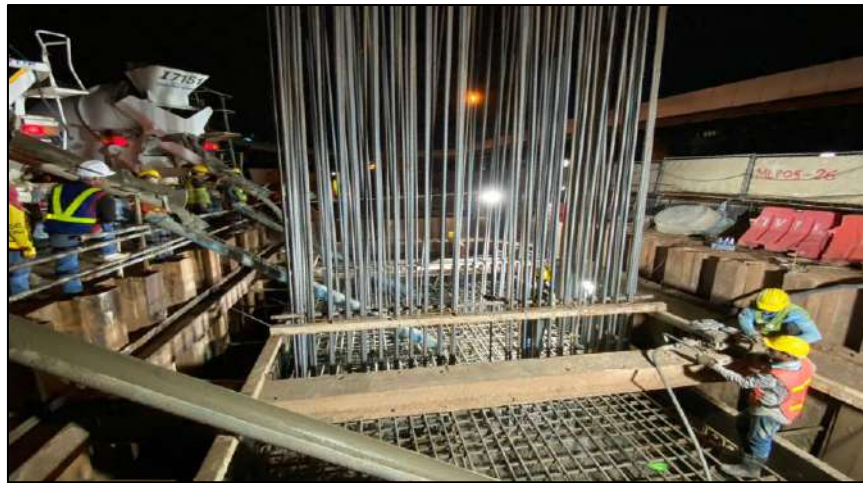
Pouring Concrete Footing 3F3.880x1.00 MLP05-26C
