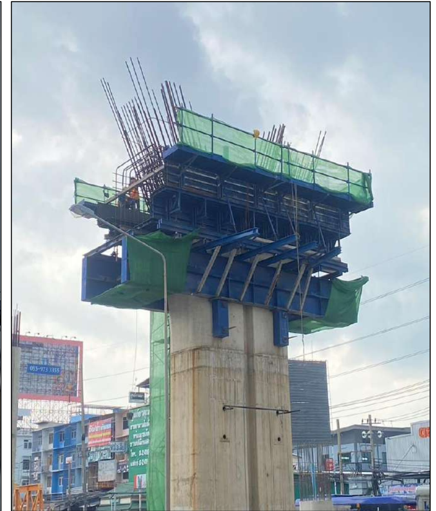
Install Steel Column Pier Type YT-1 Step LCB 8 M. MLP04-20C
