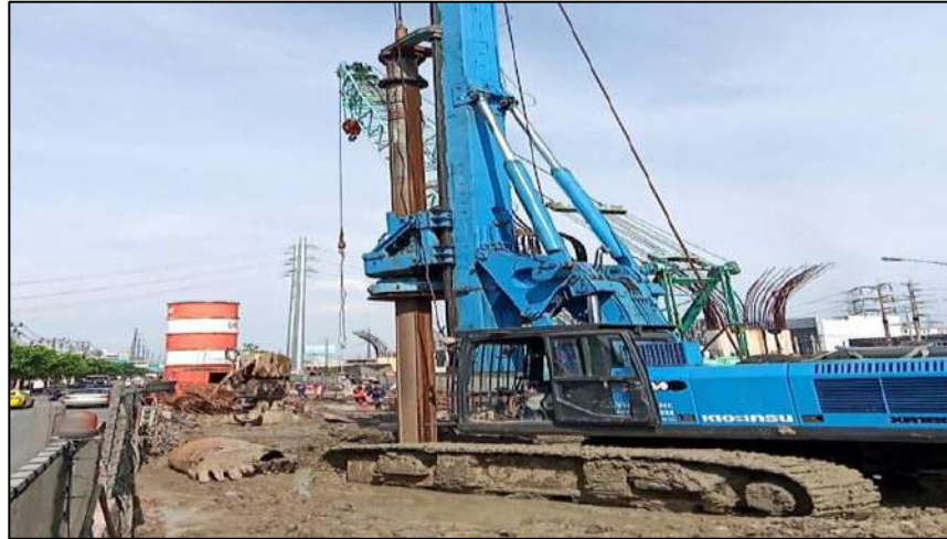
Drilling Bored Pile Dia 1.00 m. BP-5L/2
