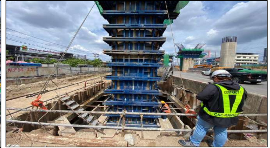
Install Steel Column Pier Type PTT-1 Step 1 MLP04-20L
