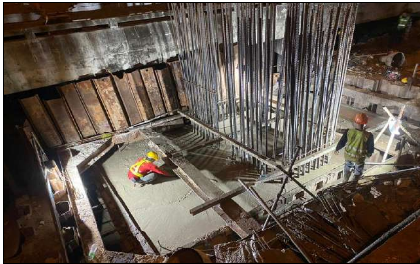
Pouring Concrete Footing 3F3.80x1.00 MLP06-07C
