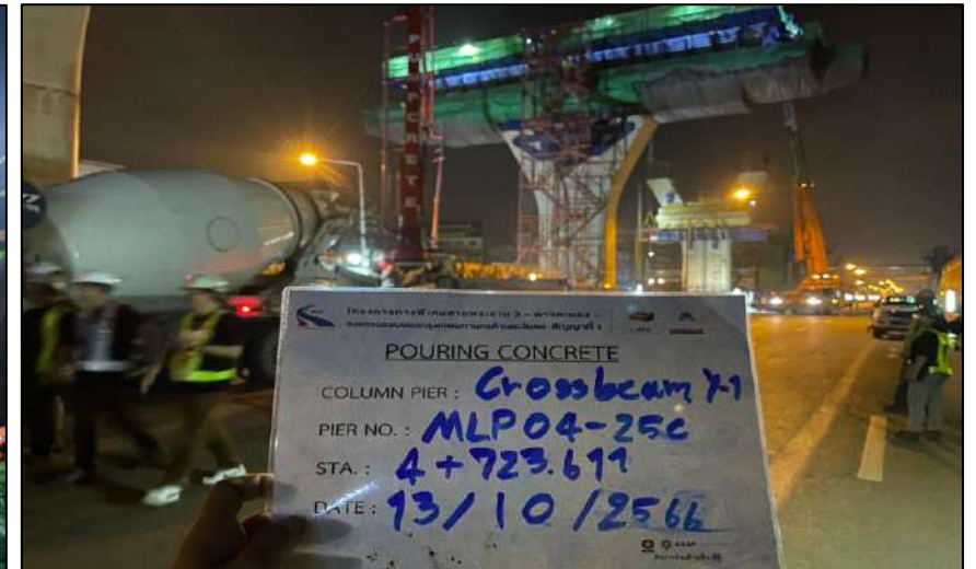
Pouring Concrete Cross Beam Pier Type Y-1 MLP04-25C
