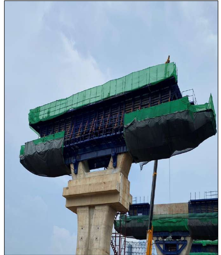
Install Steel Cross Beam Pier Type Y-1 MLP04-24C
