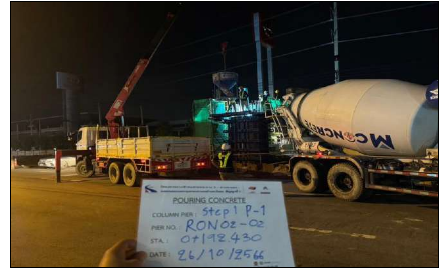
Pouring Concrete Column Pier Type P-1 Step 1 RON2-02
