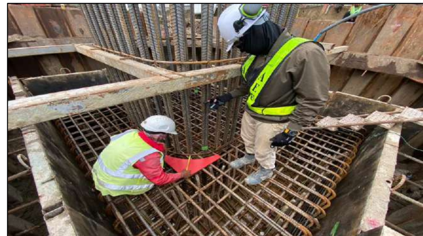
Install Steel Footing 2F3.00x1.00 MLP04-15L
