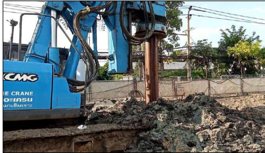
Drilling Bored Pile Dia 1.00 m. BP-3L/1
