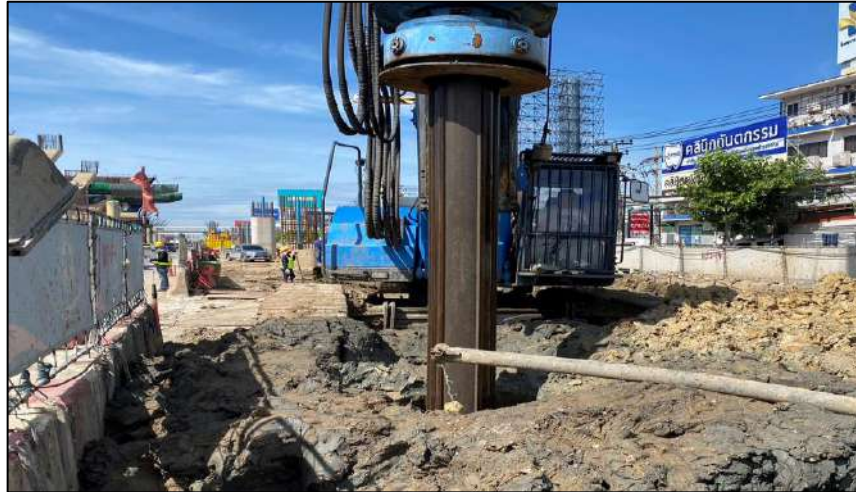
Drilling Bored Pile Dia 1.00 m. BP-1L/1
