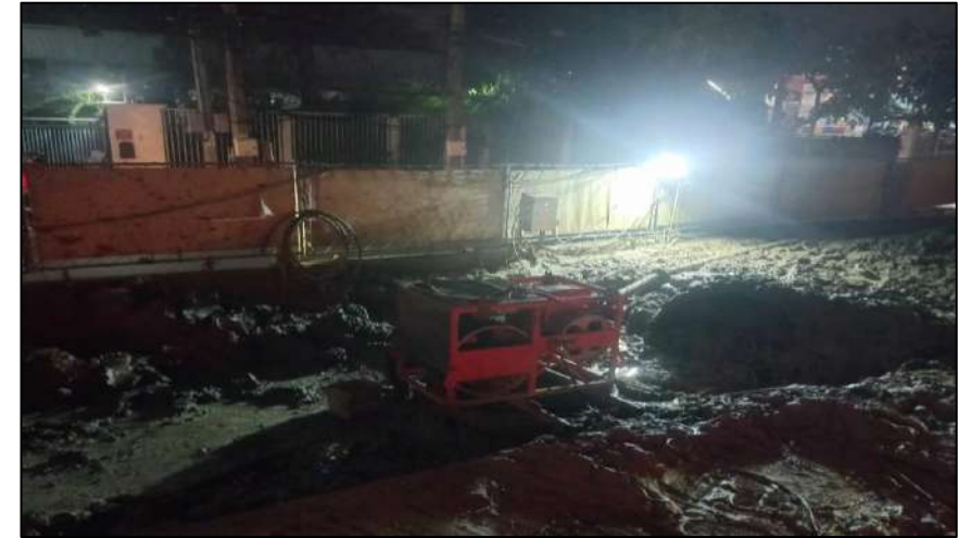
Drilling Monitor Bored Pile Test BP-3L/1
