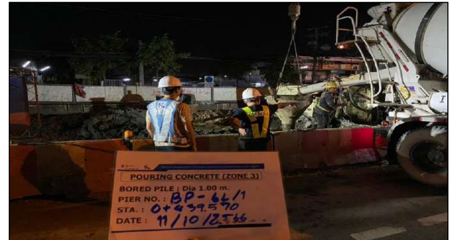
Pouring Concrete Bored Pile Dia 1.00 m. BP-6L/1
