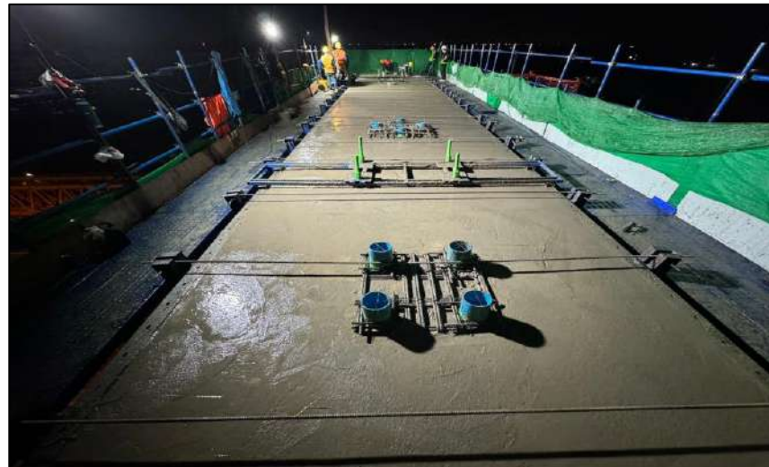
Pouring Concrete Cross Beam Pier Type Y-1 MLP04-26C
