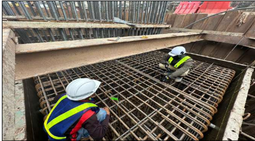
Install Steel Footing 3F3.880x1.00 MLP05-26C
