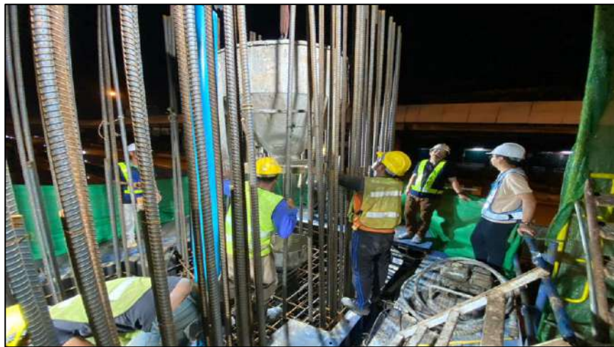
Pouring Concrete Column Pier Type Y-3 Step 1 MLP05-26C
