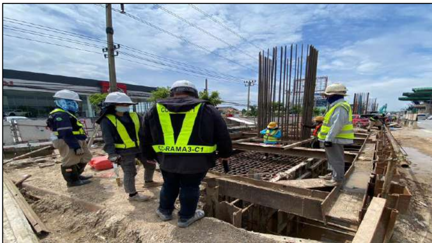
Install Steel Footing 2F3.00x1.00B RON2-02
