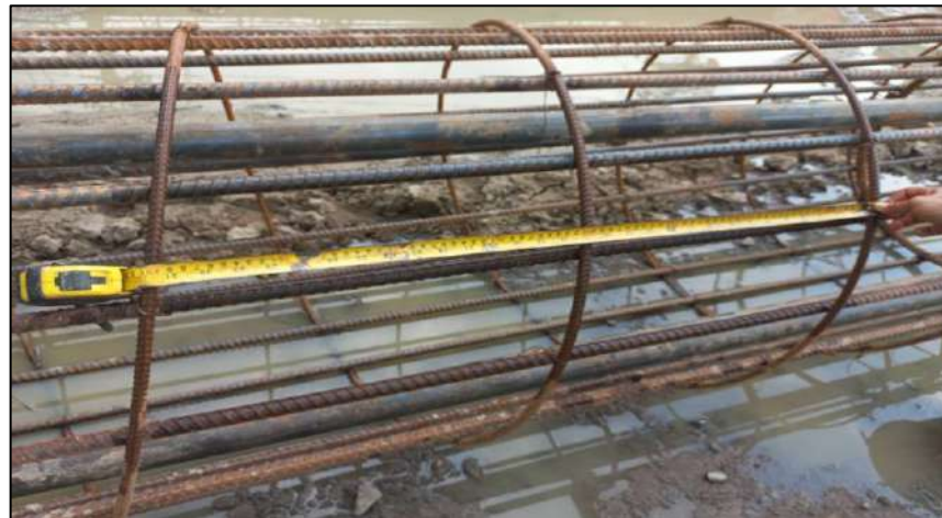
Install Rebar Bored Pile Dia 1.00 m. BP-6L/2
