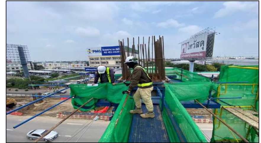
Install Steel Column Pier Type Y-1 Step Y MLP04-31C
