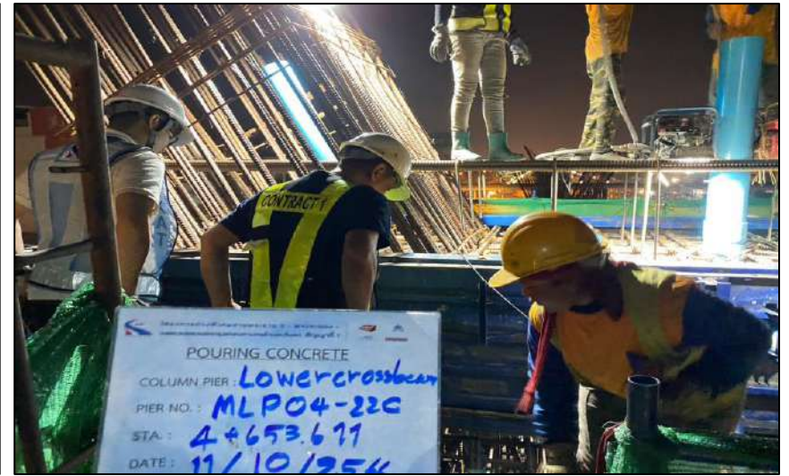
Pouring Concrete Column Pier Type YT-1 Step 3 MLP04-22C
