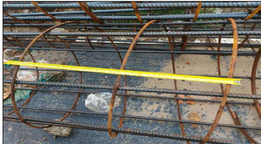
Install Rebar Bored Pile Dia 1.00 m. BP-2L/1
