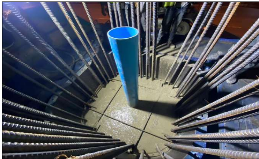
Pouring Concrete Column Pier Type P-1 Step 1 RON2-04
