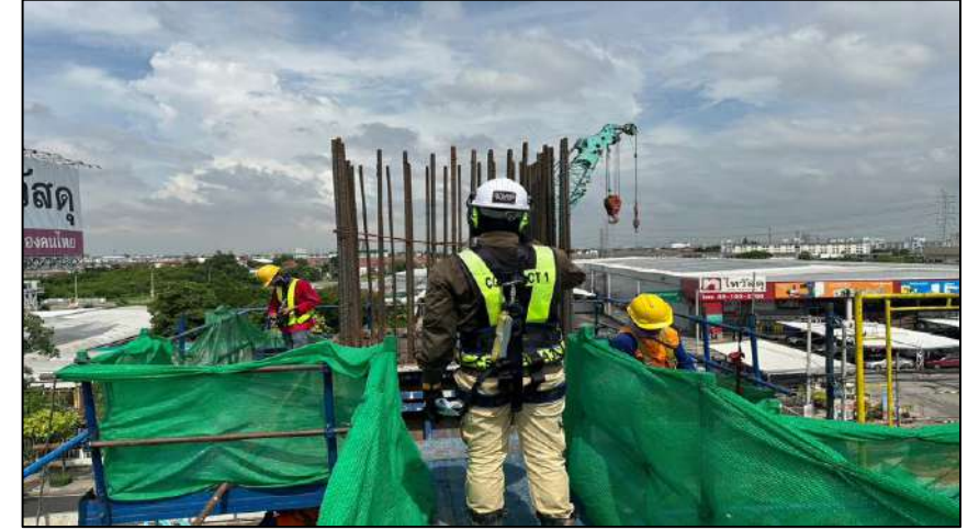
Install Steel Column Pier Type Y-1 Step Y MLP04-33C
