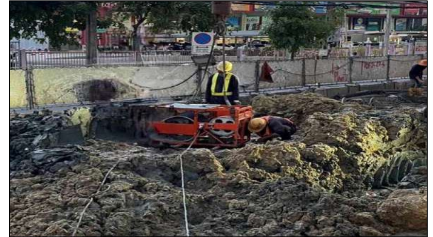
Drilling Monitor Bored Pile Test BP-5L/2
