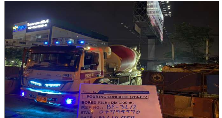
Pouring Concrete Bored Pile Dia 1.00 m. BP-3L/1
