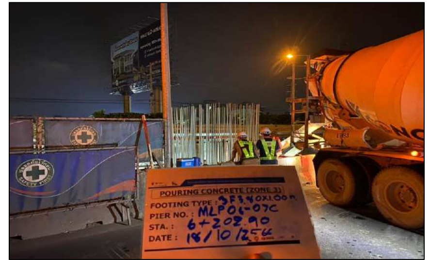
Pouring Concrete Footing 3F3.80x1.00 MLP06-07C
