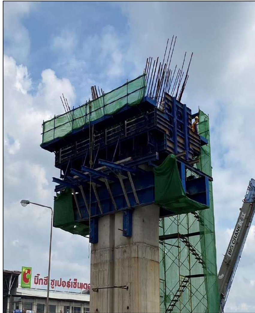
Install Steel Column Pier Type YT-1 Step LCB 8 M. MLP04-20C
