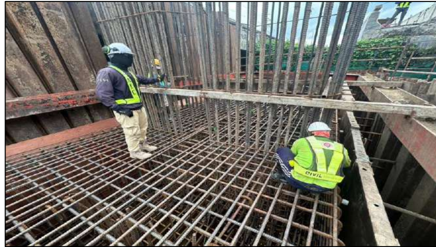
Install Steel Footing 3F3.80x1.00 MLP06-08C
