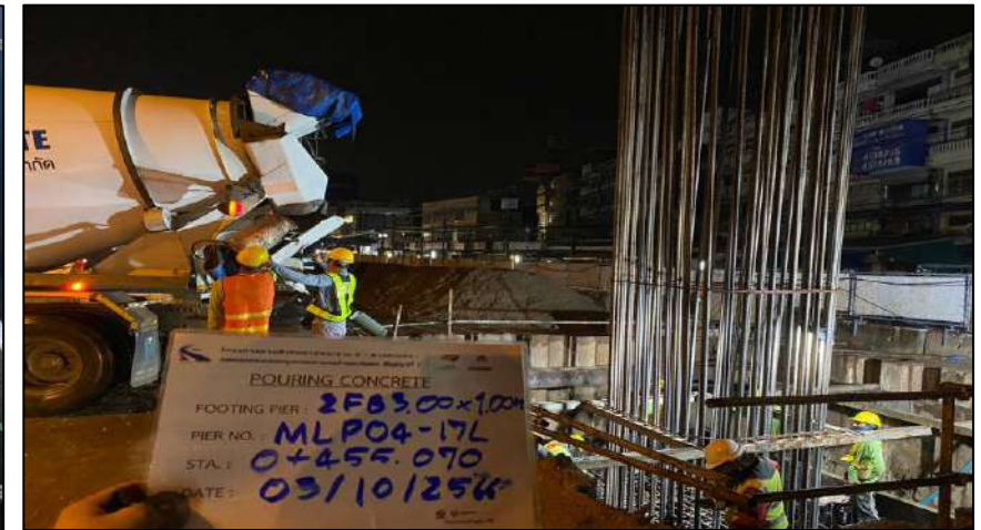
Pouring Concrete Footing 2F3.00x1.00 MLP04-17L
