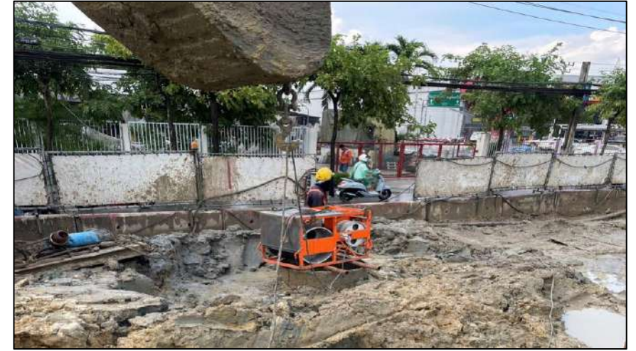
Drilling Monitor Bored Pile Test BP-4L/2
