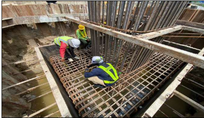
Install Steel Footing 2F3.00x1.00 MLP04-17L
