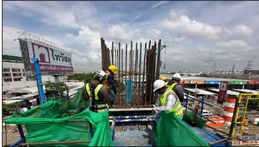
Install Steel Column Pier Type Y-1 Step Y MLP04-33C
