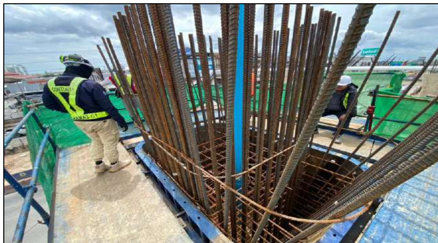
Install Steel Column Pier Type PTT-1 Step 2 MLP04-21L
