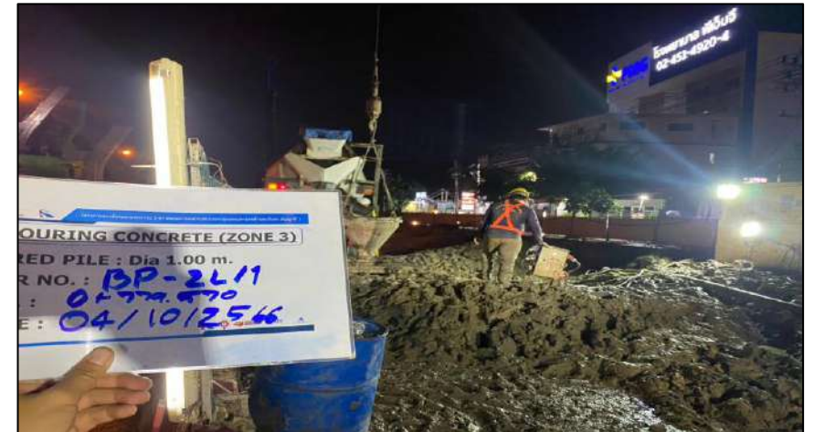
Pouring Concrete Bored Pile Dia 1.00 m. BP-2L/1
