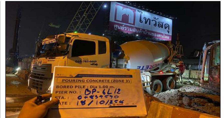
Pouring Concrete Bored Pile Dia 1.00 m. BP-6L/2
