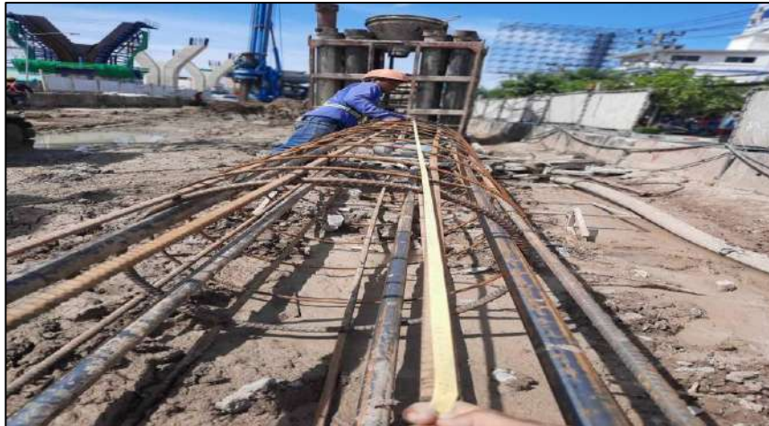
Install Rebar Bored Pile Dia 1.00 m. BP-1L/1
