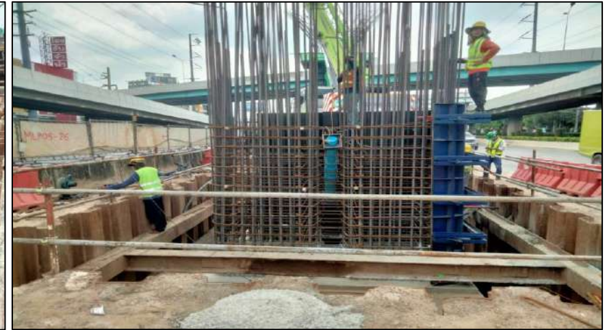
Install Steel Column Pier Type Y-3 Step 1 MLP05-26C
