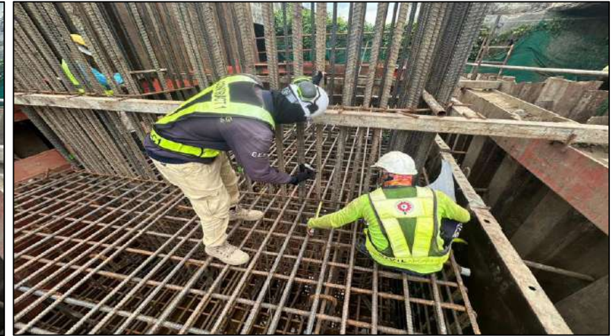
Install Steel Footing 3F3.80x1.00 MLP06-08C
