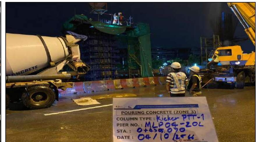
Pouring Concrete Column Pier Type PTT-1 Step 1 MLP04-20L
