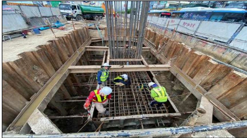
Install Steel Footing 2F3.00x1.00B MLP04-21R
