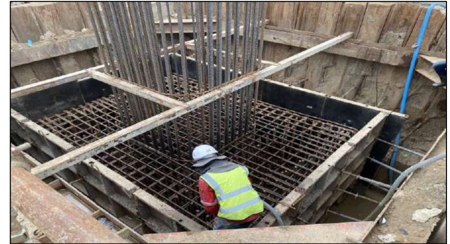
Install Steel Footing 2F3.00x1.00 ROF2-23
