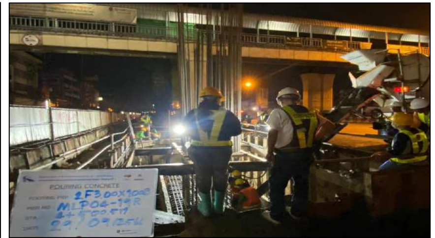
Pouring Concrete Footing 2F3.00x1.00B MLP04-19R
