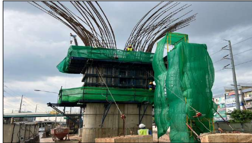
Install Steel Column Pier Type Y-3 Step 2 MLP05-25C
