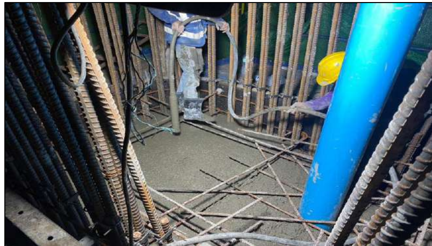
Pouring Concrete Column Pier Type Y-1 Step 1 MLP05-13C
