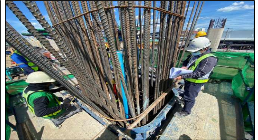
Install Steel Column Pier Type P-1 Step 2 MLP04-21L
