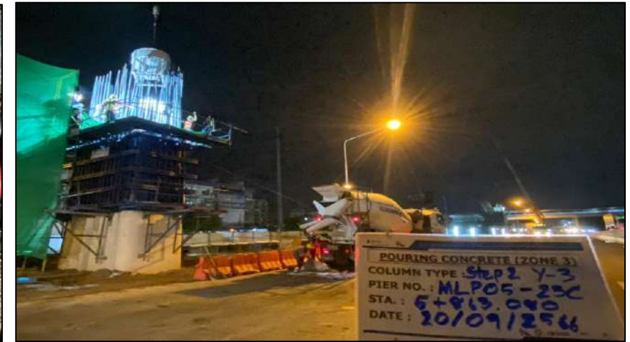
Pouring Concrete Column Pier Type Y-3 Step 2 MLP05-25C
