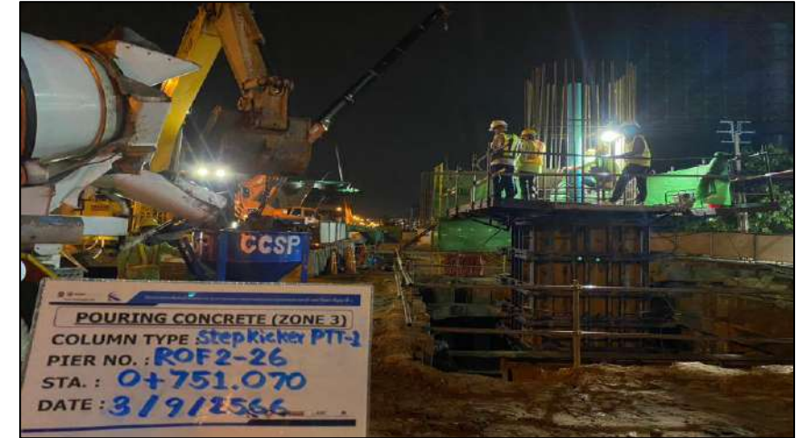
Pouring Concrete Column Pier Type P-1 Step 1 ROF2-26
