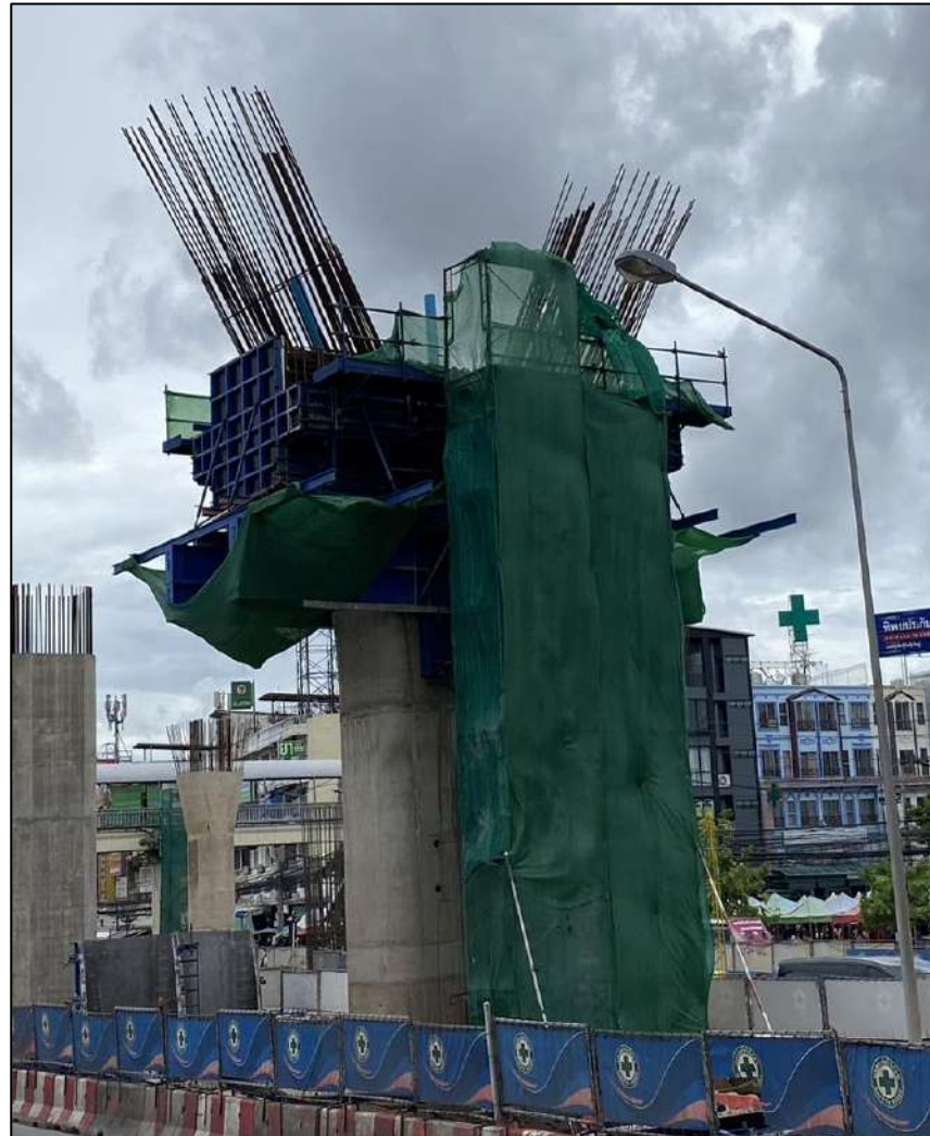
Install Steel Column Pier Type YT-2 Step 3 MLP04-22C
