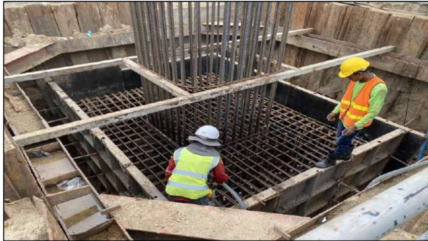
Install Steel Footing 2F3.00x1.00 ROF2-23
