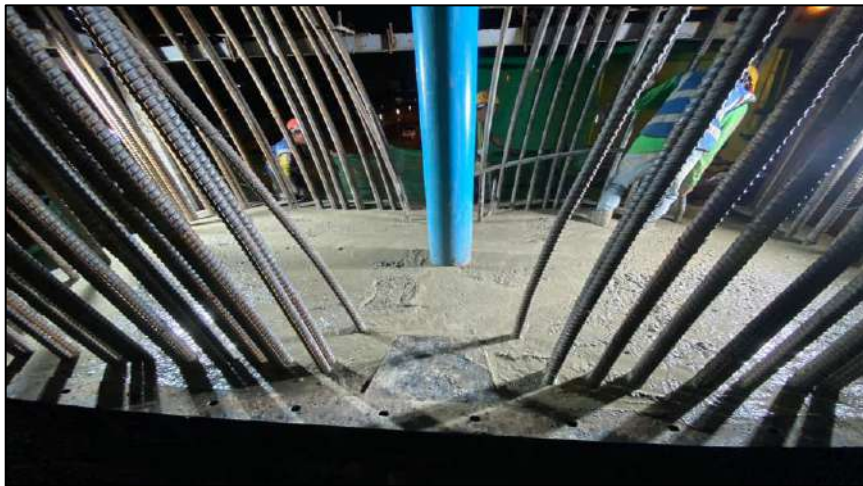
Pouring Concrete Column Pier Type Y-1 Step 2 MLP04-30C
