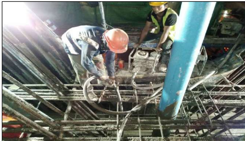
Pouring Concrete Column Pier Type YT-1 Step 3 MLP04-20C
