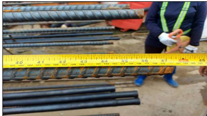
Install Rebar Bored Pile Dia 1.00 m. BP-3L/2
