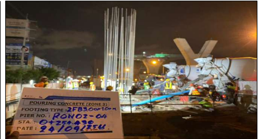
Pouring Concrete Footing 2F3.00x1.00B RON2-04
