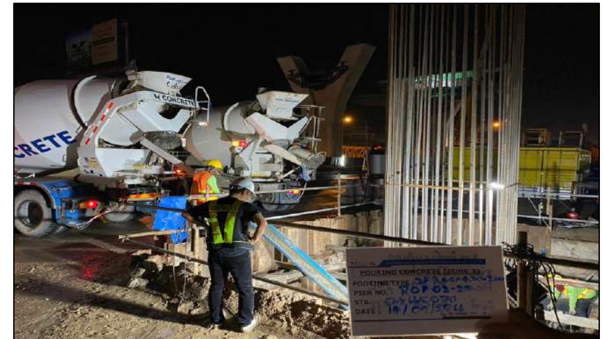
Pouring Concrete Footing 2F3.00x1.00 ROF2-23
