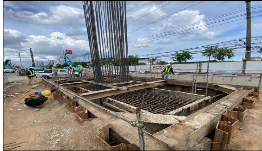
Install Steel Footing 2F3.00x1.00B RON2-03
