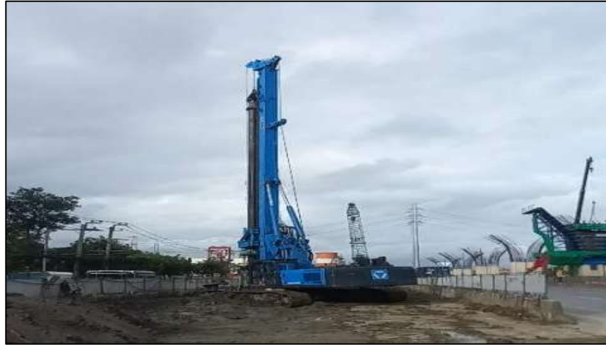
Drilling Bored Pile Dia 1.00 m. BP-3L/2
