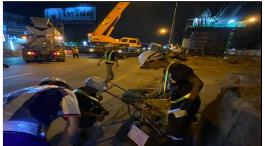
Pouring Concrete Column Pier Type Y-1 Step 2 MLP04-30C
