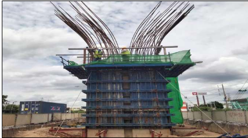
Install Steel Column Pier Type Y-1 Step 2 MLP04-30C
