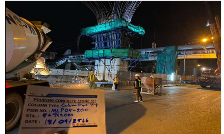
Pouring Concrete Column Pier Type Y-1 Step 2 MLP05-20C
