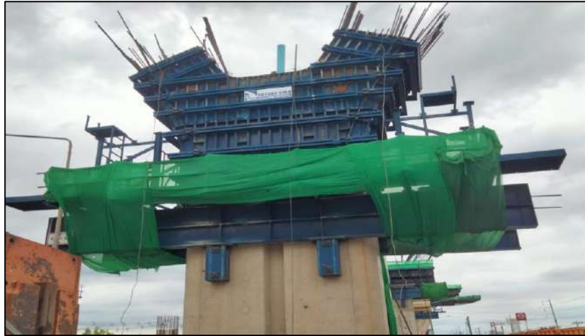
Install Steel Column Pier Type YT-1 Step 3 MLP04-20C
