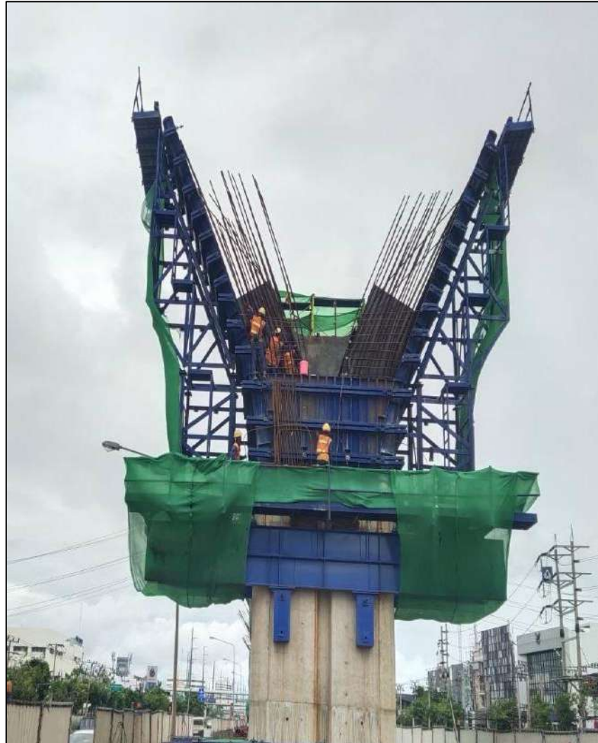
Install Steel Column Pier Type Y-1 Step Y MLP04-33C
