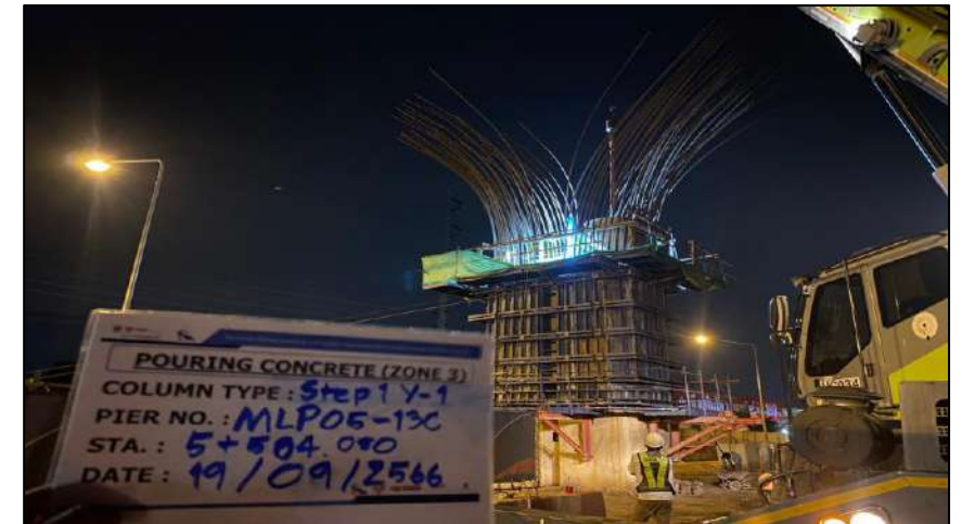
Pouring Concrete Column Pier Type Y-1 Step 1 MLP05-13C
