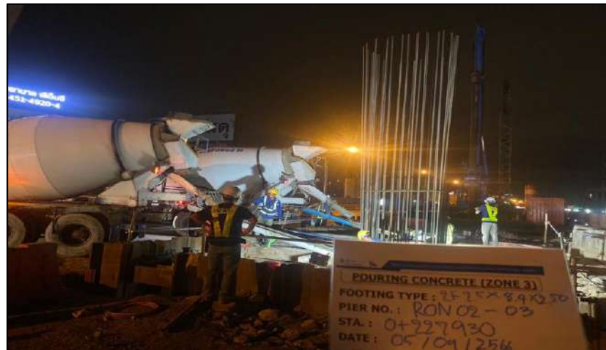
Pouring Concrete Footing 2F3.00x1.00B RON2-03
