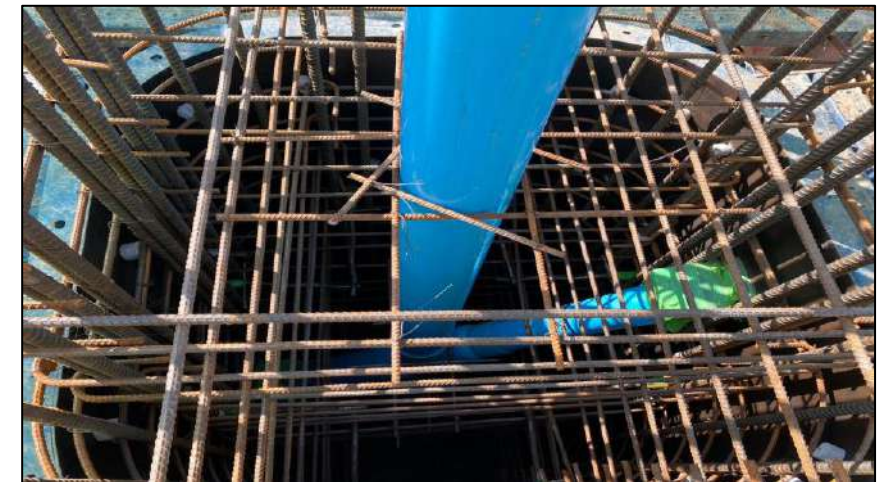
Install Steel Column Pier Type P-1 Step 1 ROF2-26
