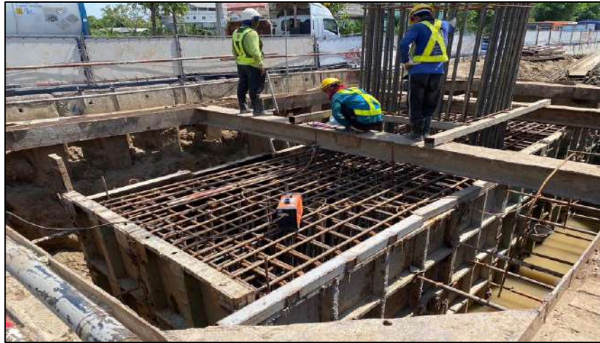
Install Steel Column Footing 2F3.00x1.00B RON2-04
