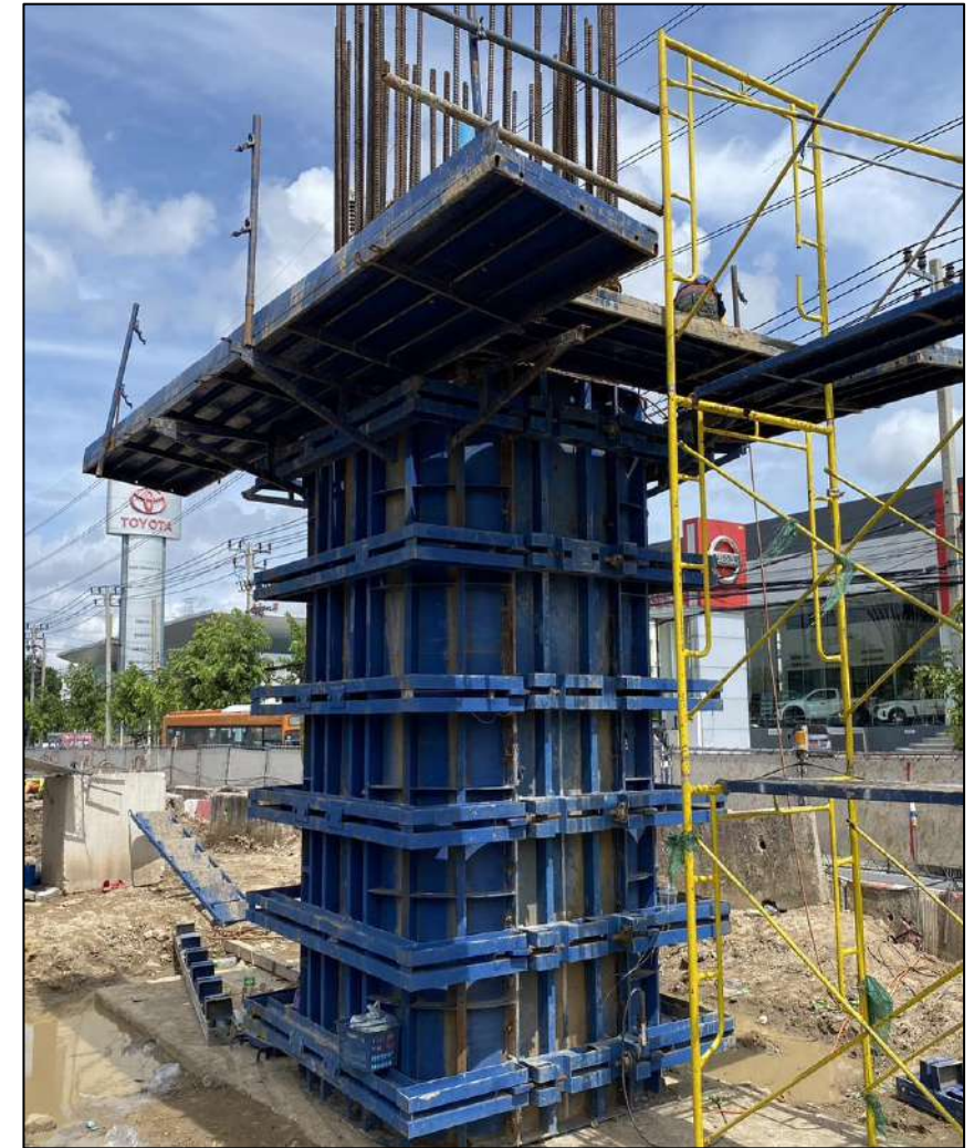
Install Steel Column Pier Type P-1 Step 1 RON2-03
