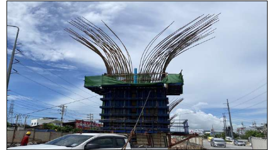
Install Steel Column Pier Type Y-1 Step 1 MLP05-13C
