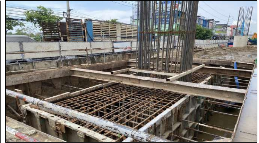
Install Steel Column Footing 2F3.00x1.00B RON2-04
