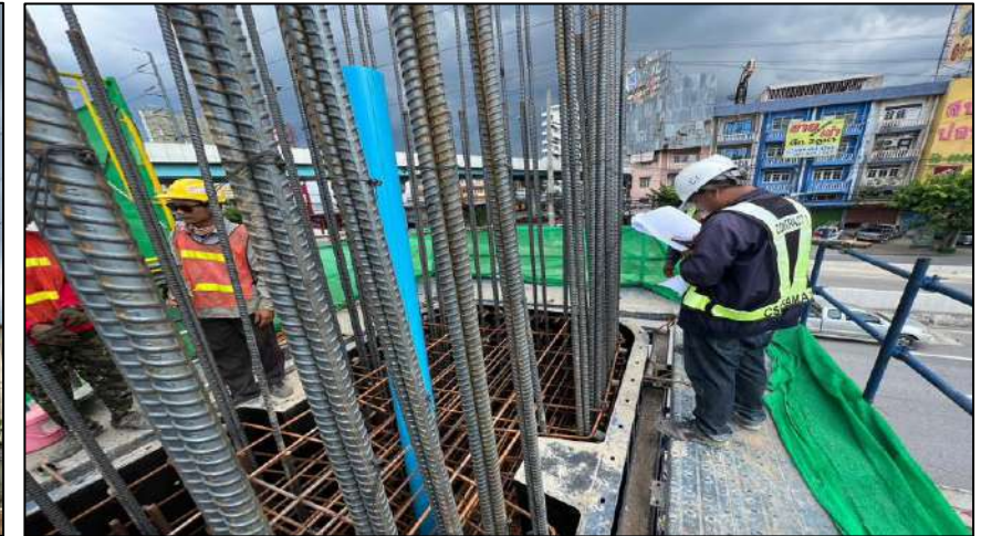
Install Steel Column Pier Type Y-3 Step 2 MLP05-25C
