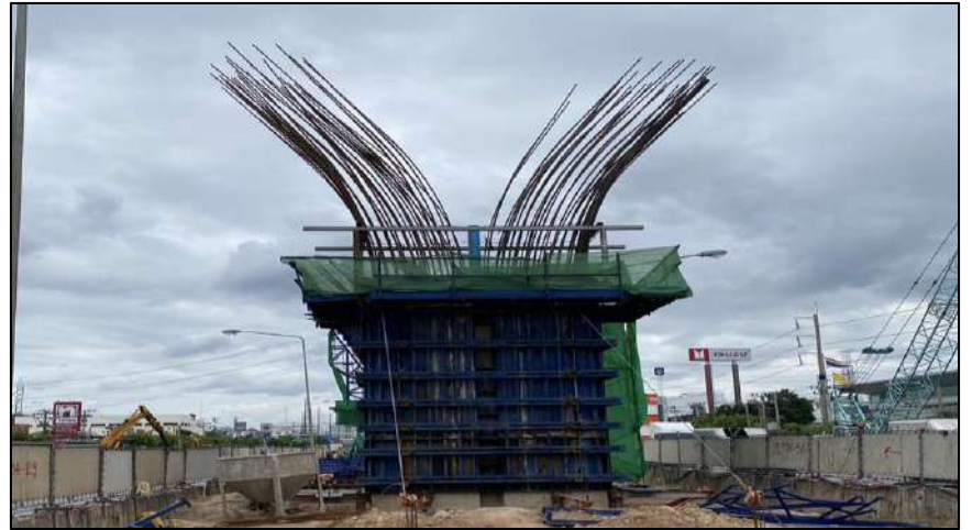
Install Steel Column Pier Type Y-1 Step 2 MLP04-30C
