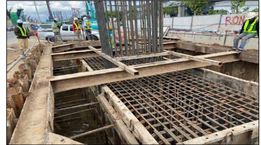
Install Steel Footing 2F3.00x1.00B RON2-03
