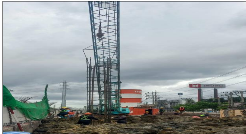
Install Rebar Bored pile Dia 1.00 m. BP-1R/2
