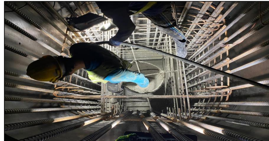
Pouring Concrete Column Pier Type PTT-1 Step 1 MLP04-22L
