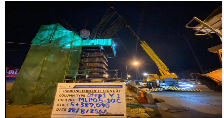
Pouring Concrete Column Pier Type Y-1 Step 2 MLP05-10C
