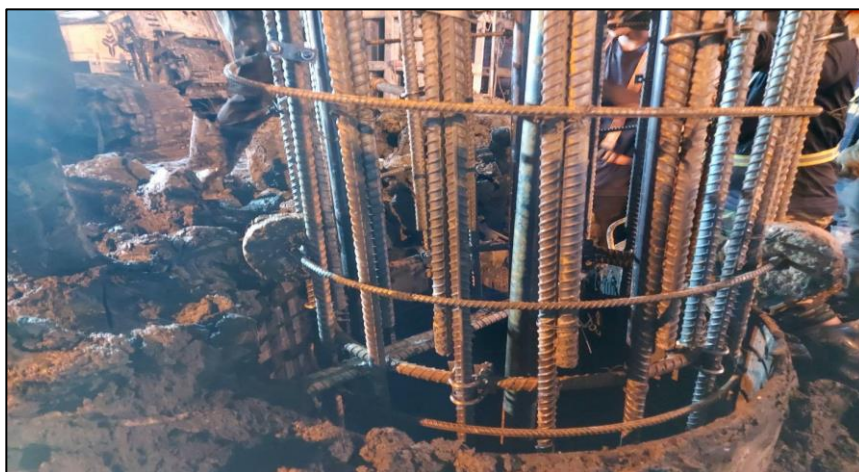
Install Rebar Bored pile Dia 1.00 m. BP-5R/2
