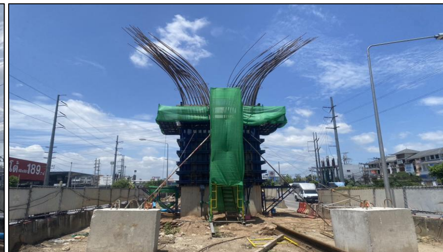
Install Steel Column Pier Type Y-1 Step 2 MLP05-11C
