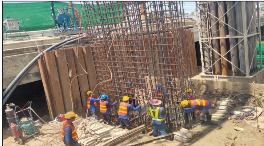
Install Rebar Barrette pile 3.80x1.00 m. MLP06-08C/3
