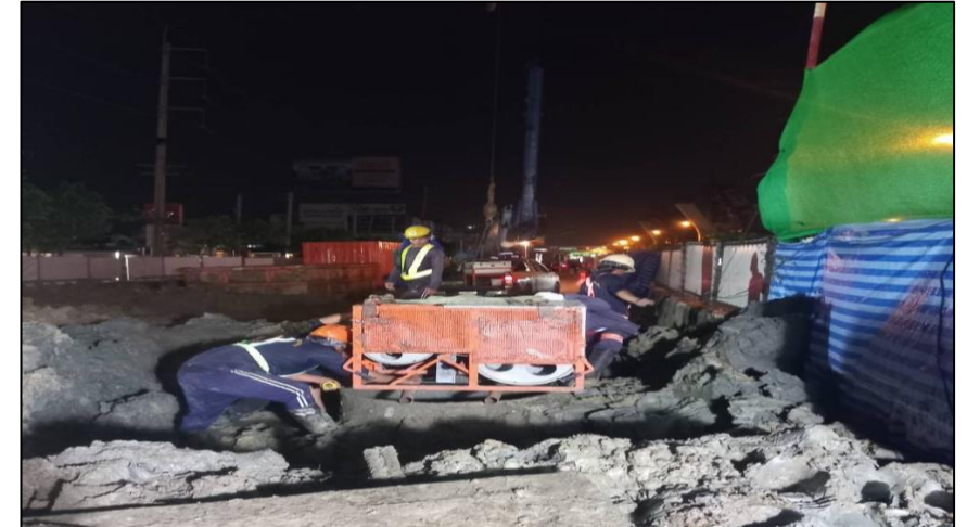
Drilling monitor Test BP-1R/2
