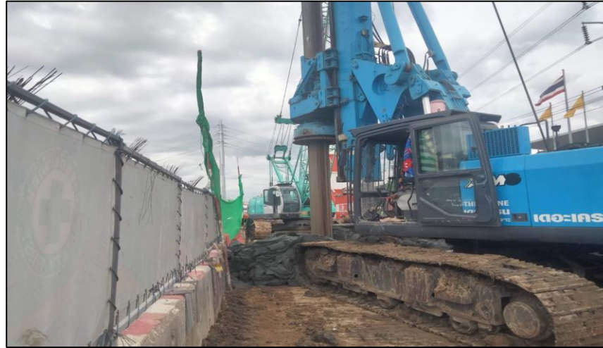
Grabbing Bored pile Dia 1.00 m. BP-4R/2
