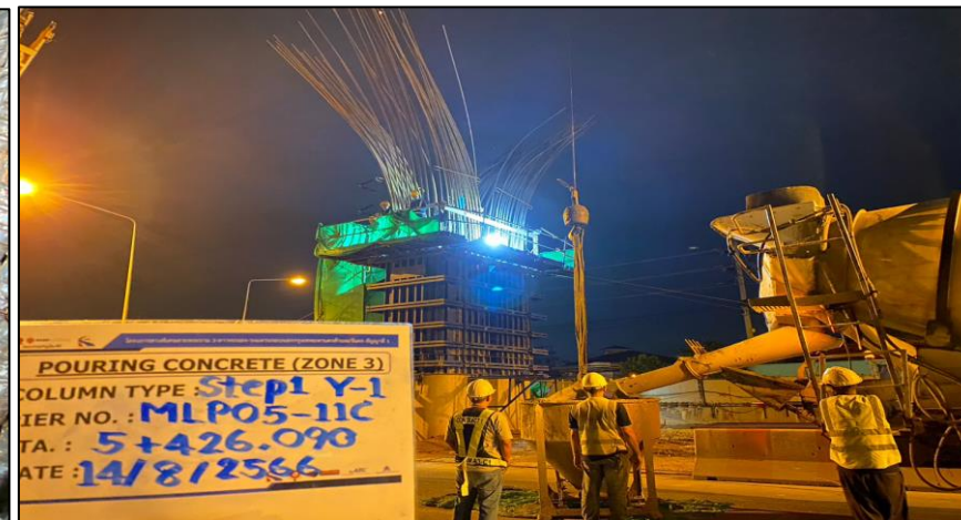
Pouring Concrete Column Pier Type Y-1 Step 2 MLP05-11C
