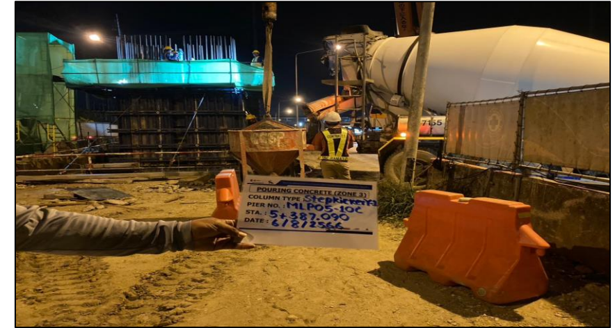
Pouring Concrete Column Pier Type Y-1 Step 1 MLP05-10C
