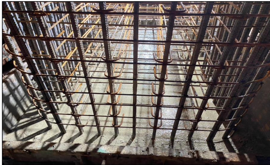
Pouring Concrete Column Pier Type Y-3 Step 1 MLP05-25C
