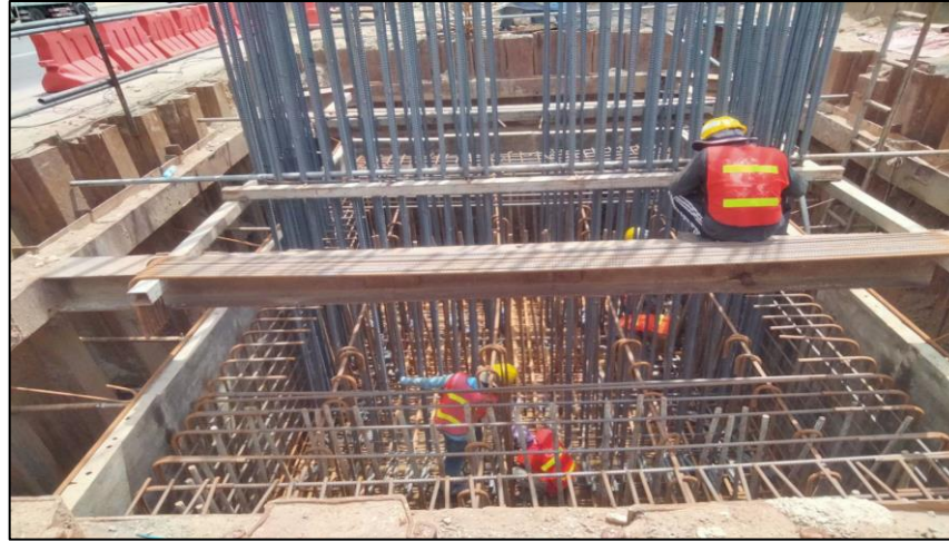
Install Steel Footing 3F3.80x1.00 m. MLP05-25C
