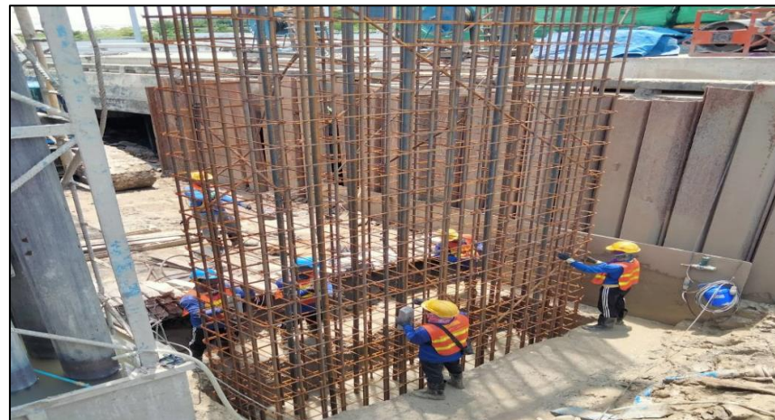
Install Rebar Barrette pile 3.80x1.00 m. MLP06-08C/1
