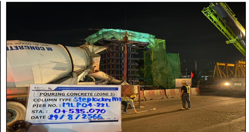
Pouring Concrete Column Pier Type PTT-1 Step 1 MLP04-22L
