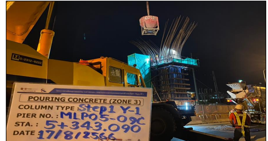
Pouring Concrete Column Pier Type Y-1 Step 2 MLP05-09C
