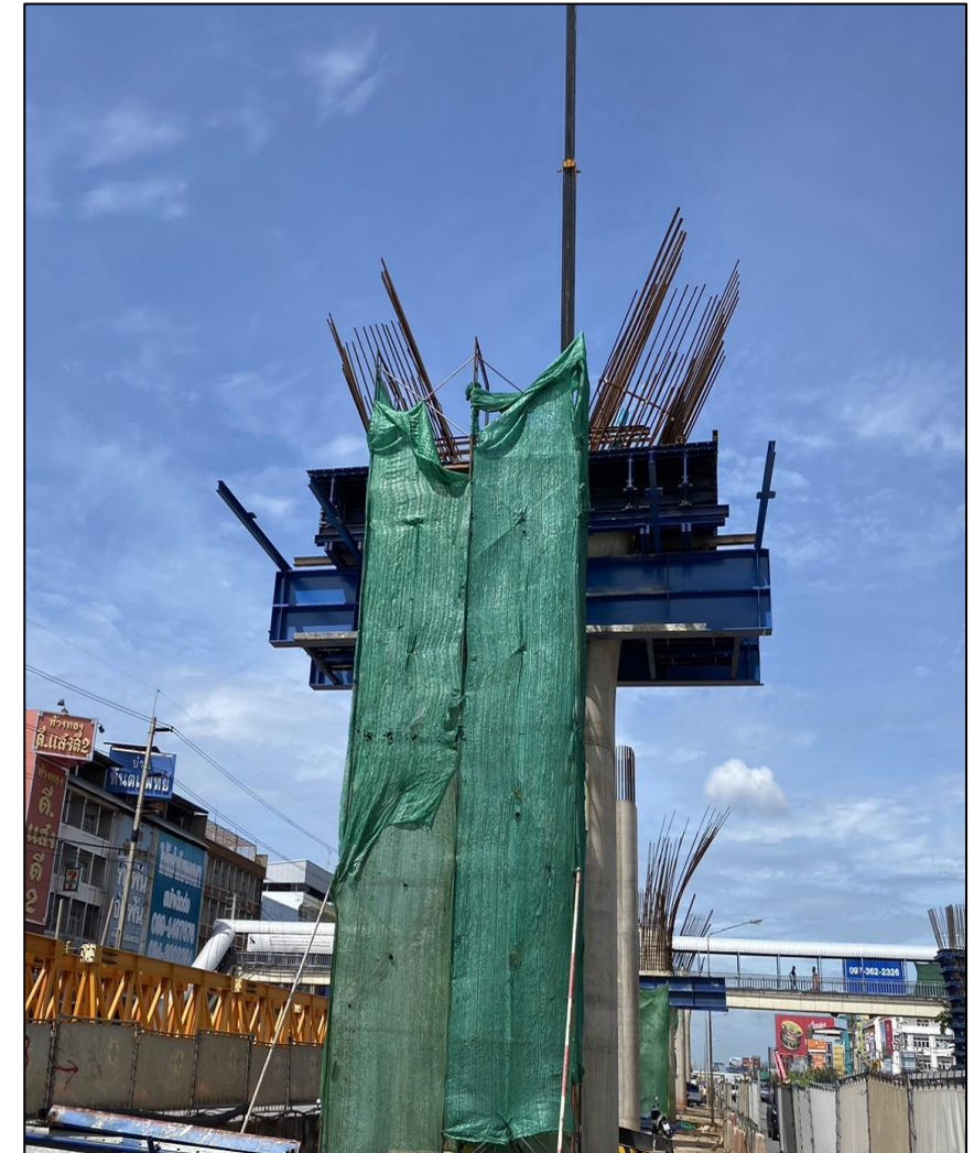
Pouring Concrete Column Pier Type YT-2 Step 3 MLP04-22C
