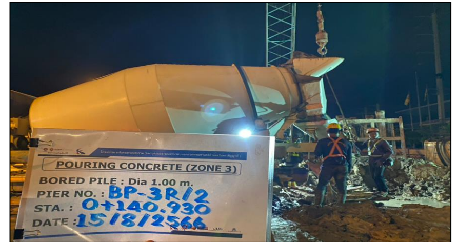
Pouring concrete Bored pile Dia 1.00 m. BP-3R/2
