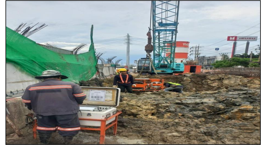
Drilling monitor Test BP-3R/2
