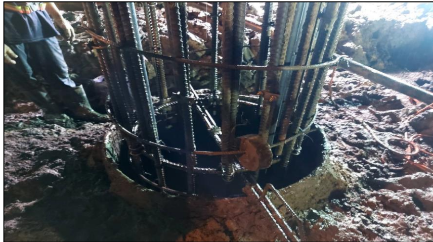
Install Rebar Bored pile Dia 1.00 m. BP-4R/2
