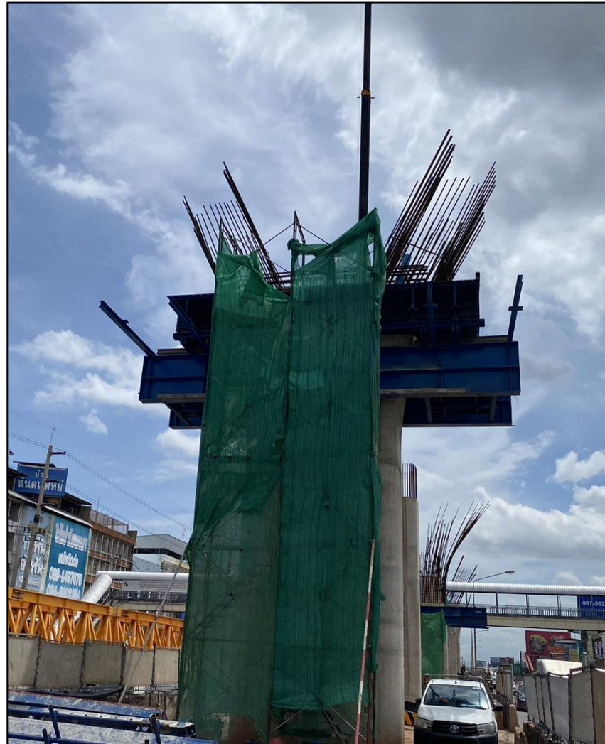
Pouring Concrete Column Pier Type YT-2 Step 3 MLP04-22C
