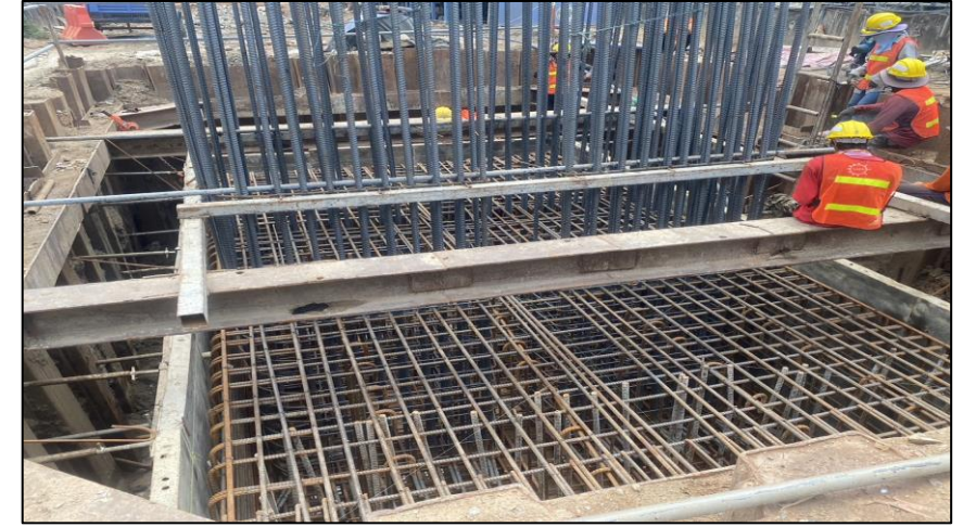
Install Steel Footing 3F3.80x1.00 m. MLP05-25C
