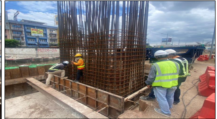
Install Steel Column Pier Type Y-3 Step 1 MLP05-23C
