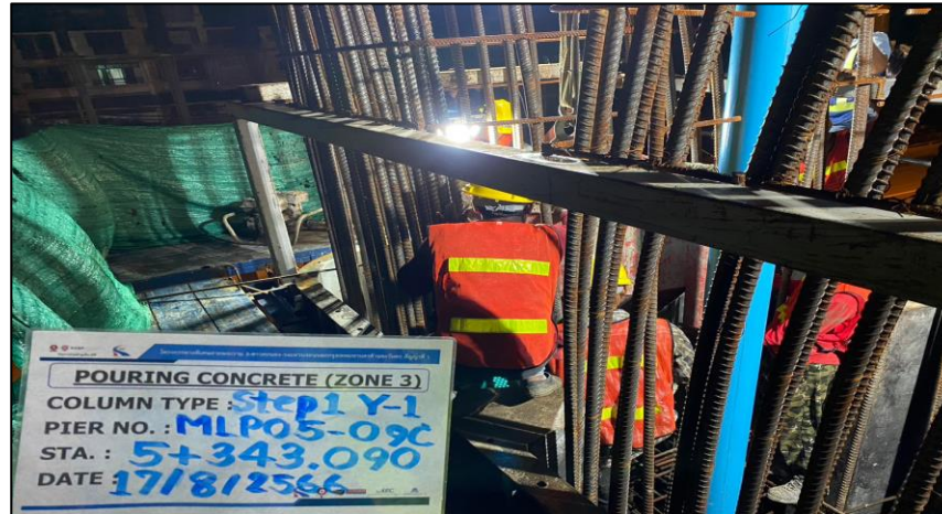
Pouring Concrete Column Pier Type Y-1 Step 2 MLP05-09C
