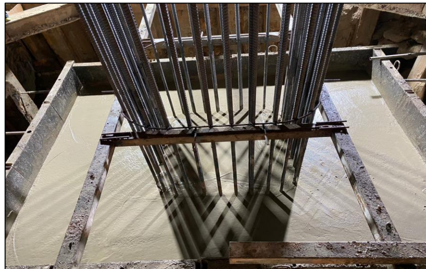
Pouring Concrete Footing 2F3.00x1.00 m. ROF2-25
