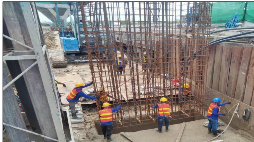
Install Rebar Barrette pile 3.80x1.00 m. MLP06-08C/2
