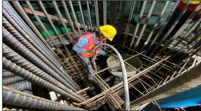
Pouring Concrete Column Pier Type Y-1 Step 1 MLP05-10C
