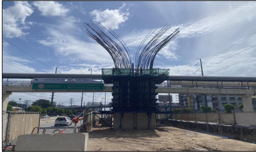
Install Steel Column Pier Type Y-1 Step 2 MLP05-19C
