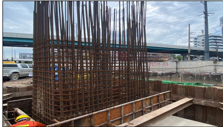
Install Steel Column Pier Type Y-3 Step 1 MLP05-23C
