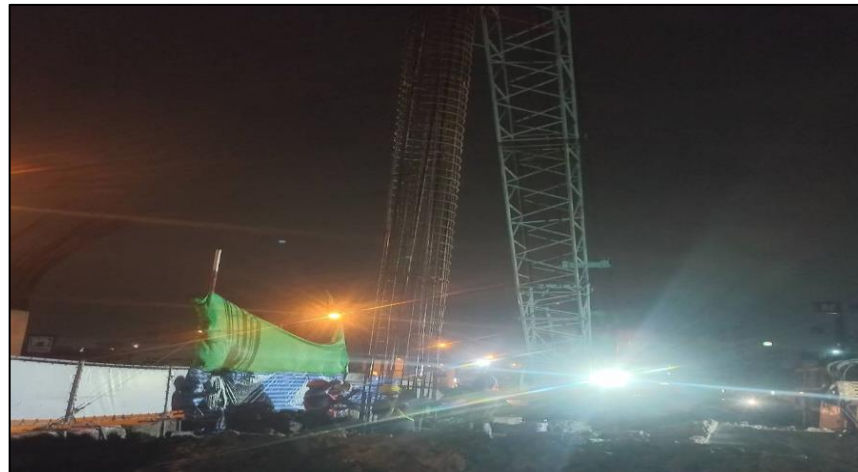
Install Rebar Bored pile Dia 1.00 m. BP-2R/2
