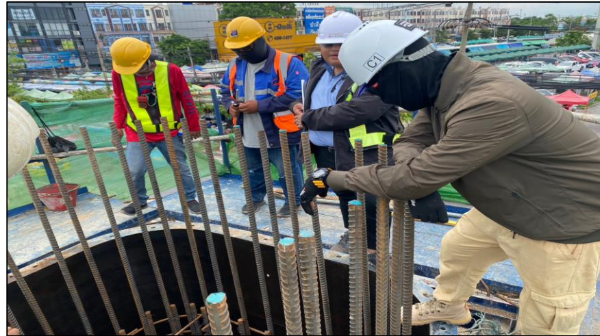
Install Steel Column Pier Type PTT-1 Step 1 MLP04-22L
