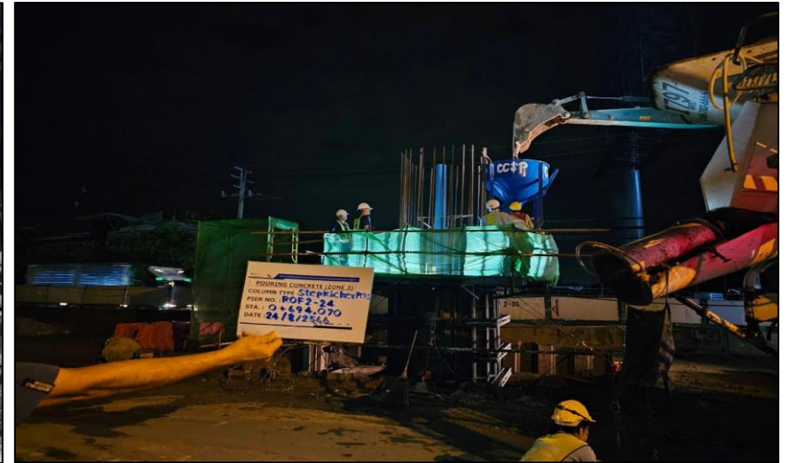
Pouring Concrete Column Pier Type P-1 Step 1 ROF2-24
