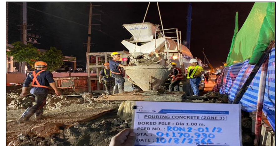
Pouring concrete Bored Pile Dia 1.00 m. RON2-01/2
