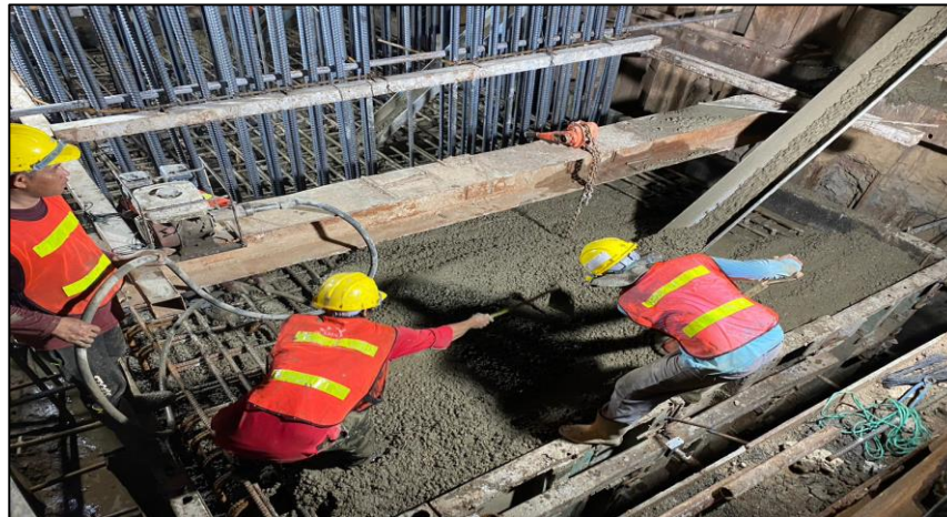
Pouring Concrete Footing 3F3.80x1.00 m. MLP05-25C
