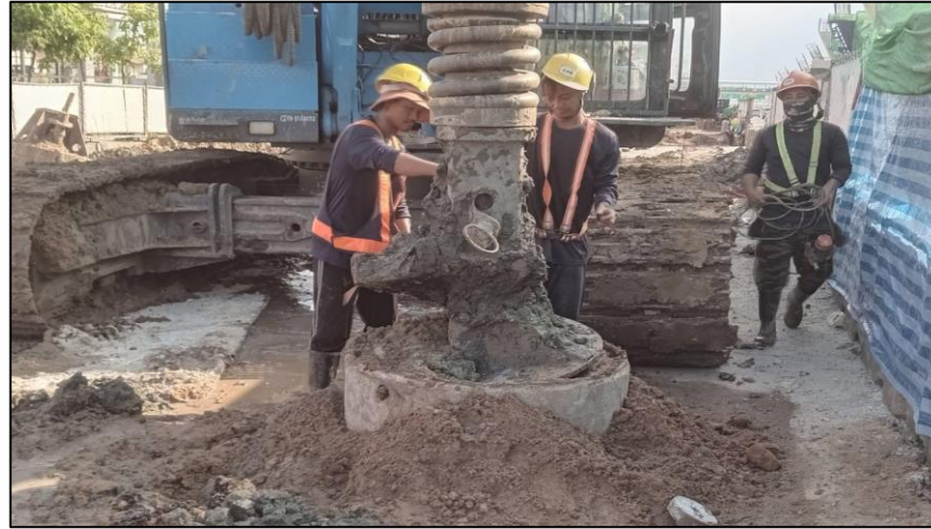
Grabbing Bored pile Dia 1.00 m. BP-2R/2
