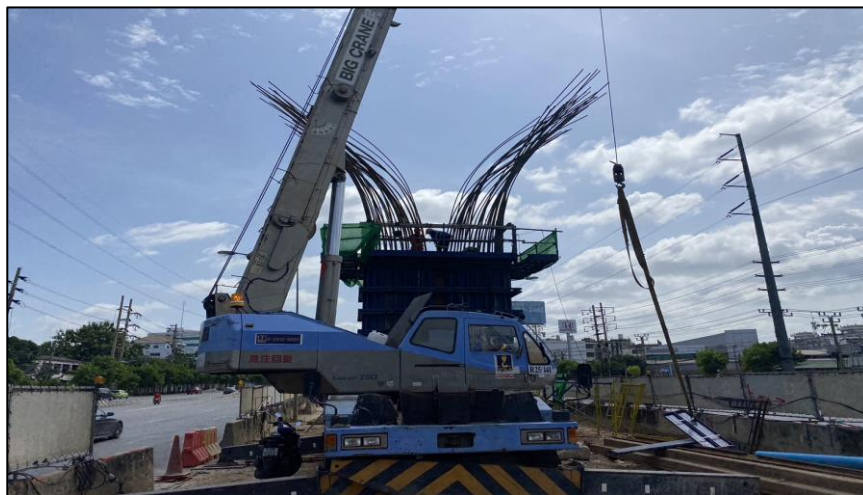
Install Steel Column Pier Type Y-1 Step 2 MLP05-11C
