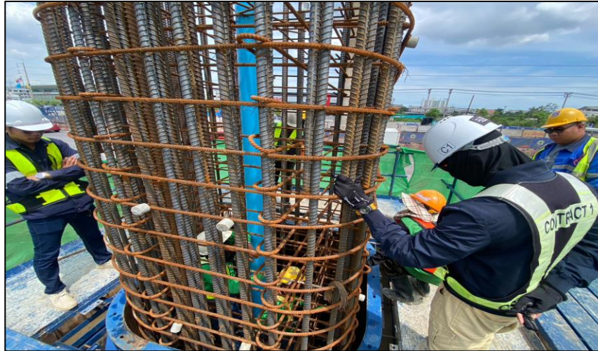
Install Steel Column Pier Type P-1 Step 1 ROF2-25
