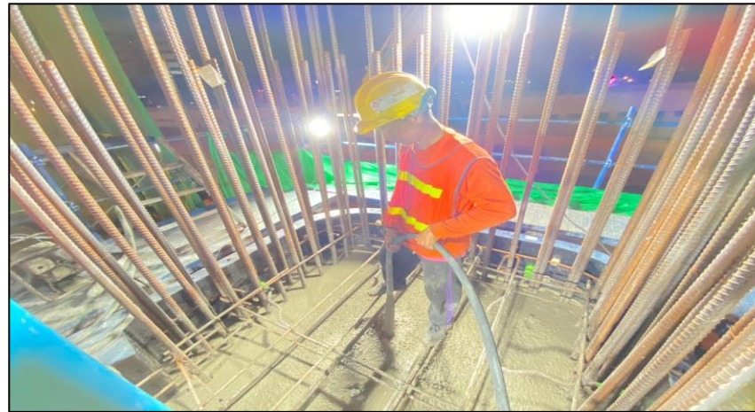
Pouring Concrete Column Pier Type Y-1 Step 2 MLP05-10C
