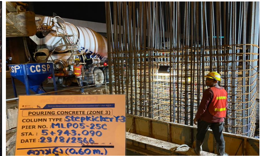
Pouring Concrete Column Pier Type Y-3 Step 1 MLP05-25C
