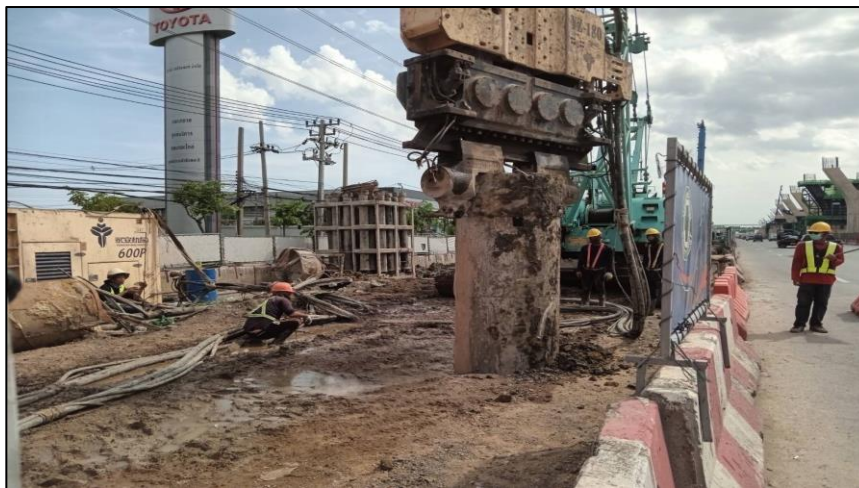
Grabbing Bored pile Dia 1.00 m. BP-5R/2
