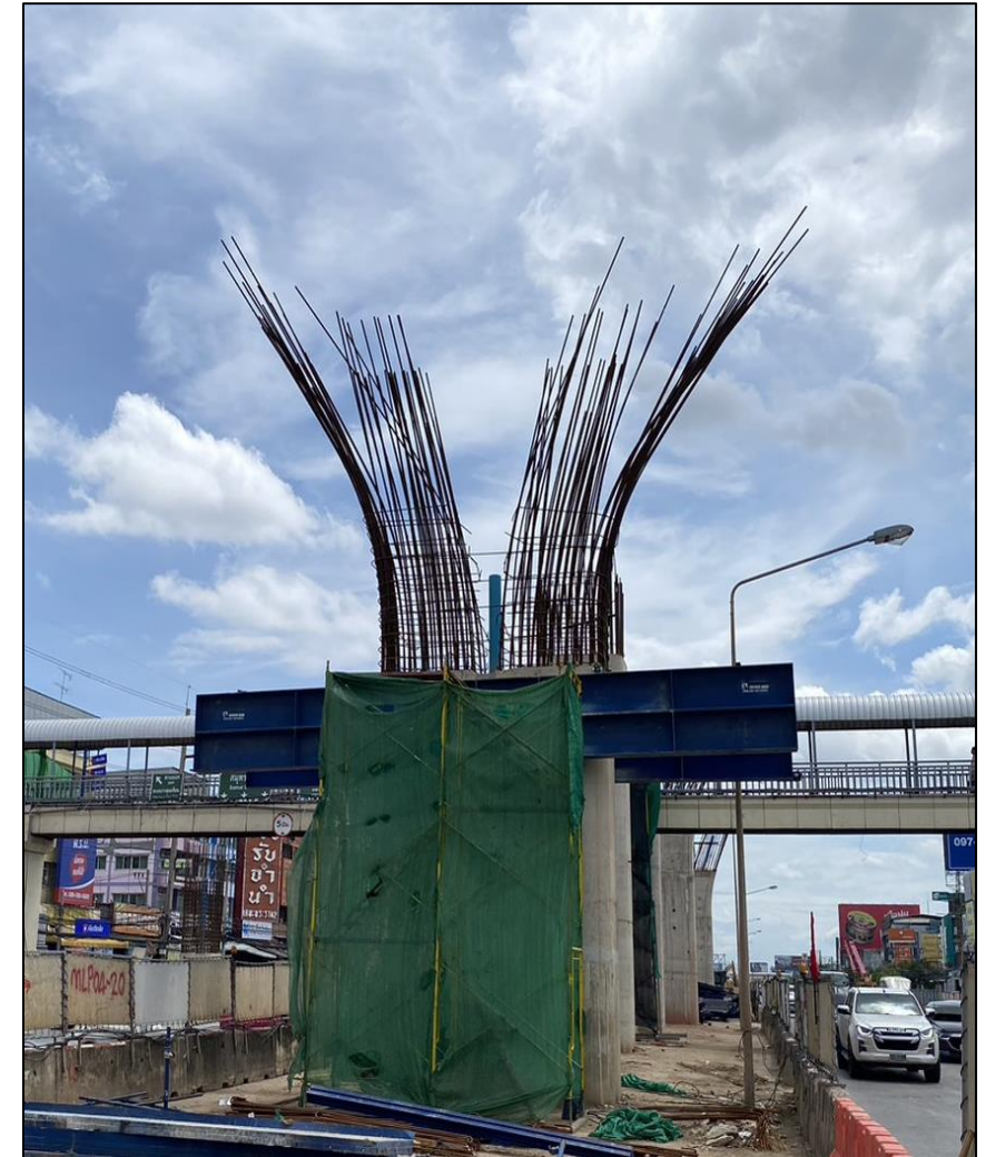
Install Steel Column Pier Type Y-1 Step Y MLP04-20C
