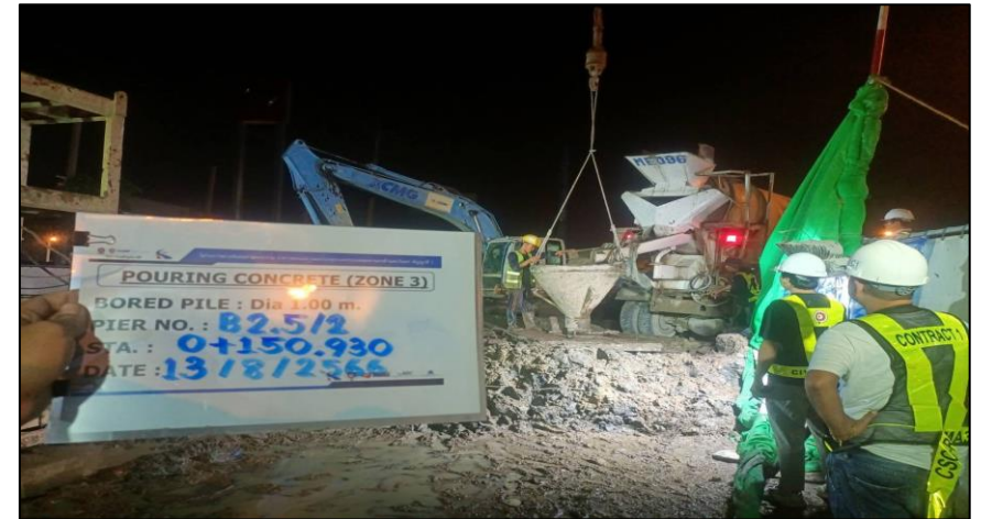
Pouring concrete Bored pile Dia 1.00 m. BP-2R/2
