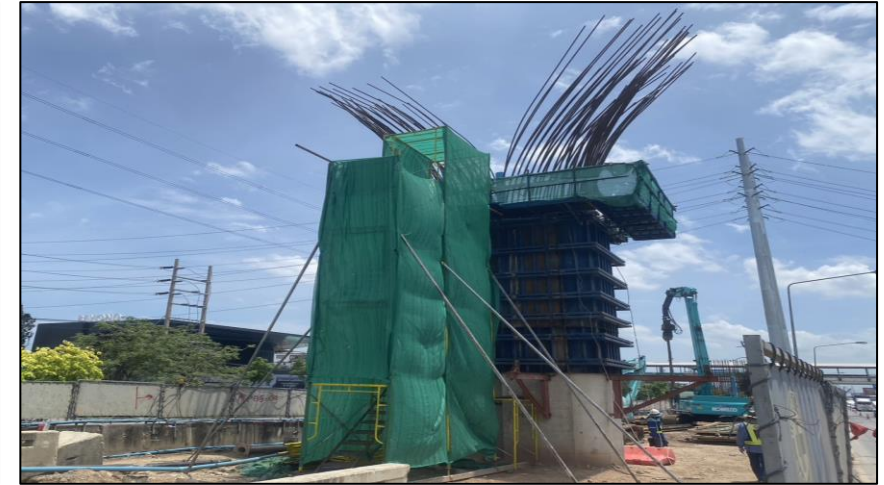
Install Steel Column Pier Type Y-1 Step 2 MLP05-09C
