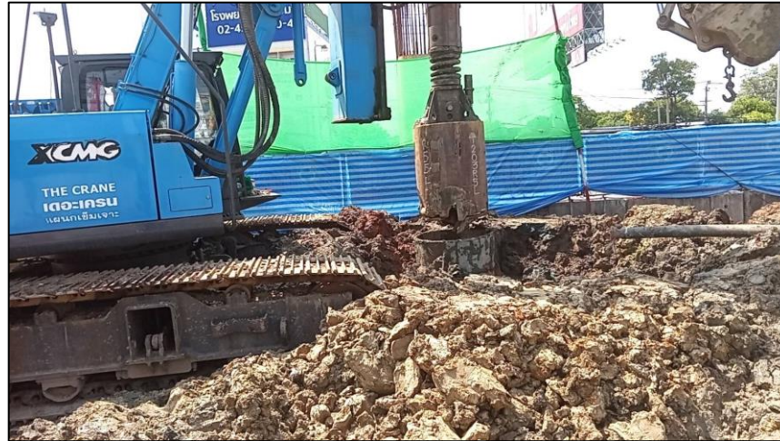
Grabbing Bored Pile Dia 1.00 m. RON2-01/2
