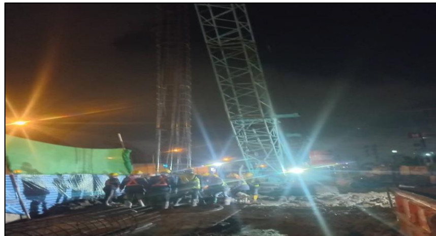
Install Rebar Bored Pile Dia 1.00 m. RON2-01/2
