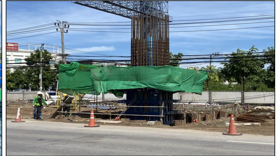
Install Steel Column Pier Type P-1 Step 1 ROF2-25
