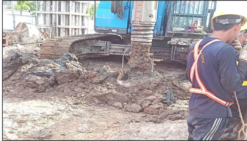
Grabbing Bored pile Dia 1.00 m. BP-3R/2
