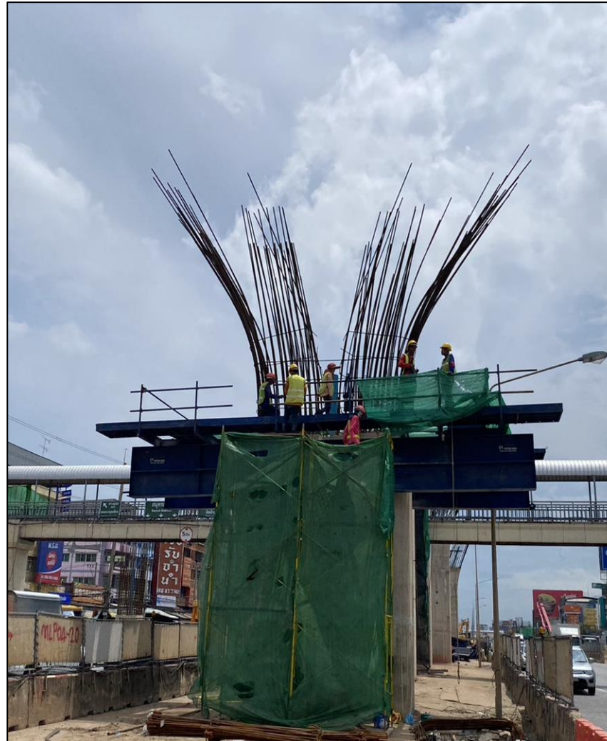
Install Steel Column Pier Type Y-1 Step Y MLP04-20C
