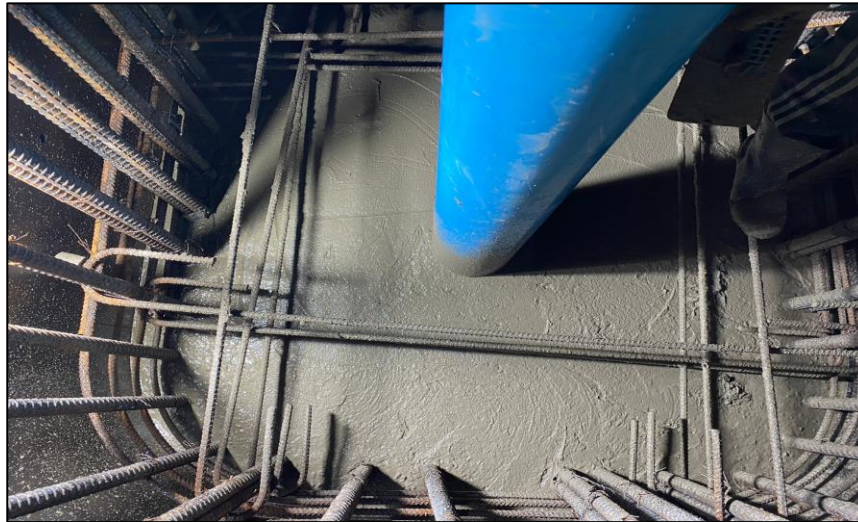
Pouring Concrete Column Pier Type P-1 Step 1 ROF2-24
