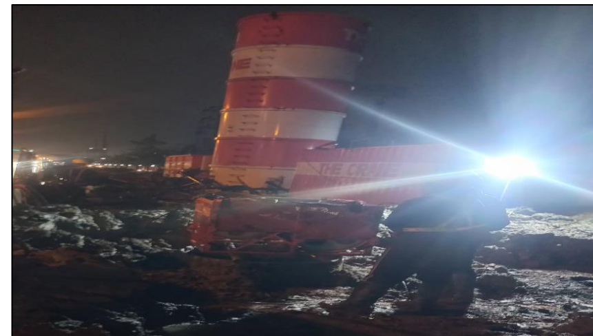
Drilling monitor Test BP-5R/2
