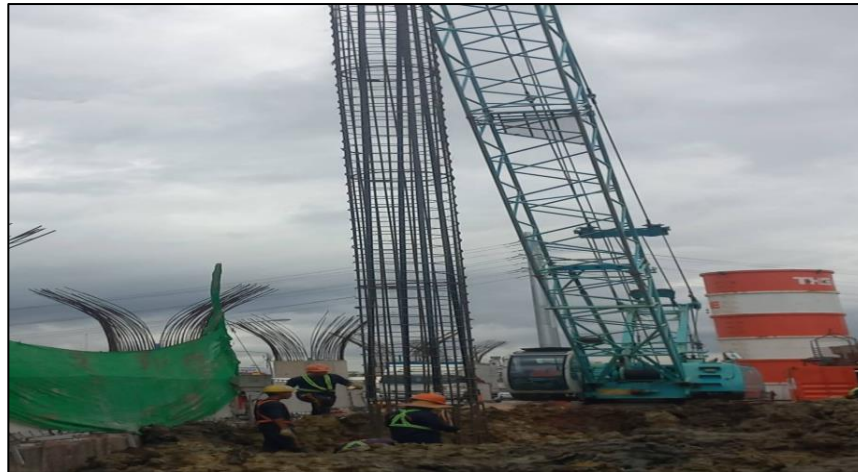
Install Rebar Bored pile Dia 1.00 m. BP-3R/2
