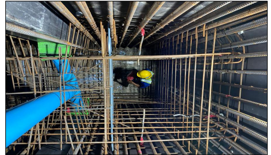
Install Steel Column Pier Type Y-1 Step 2 MLP05-19C
