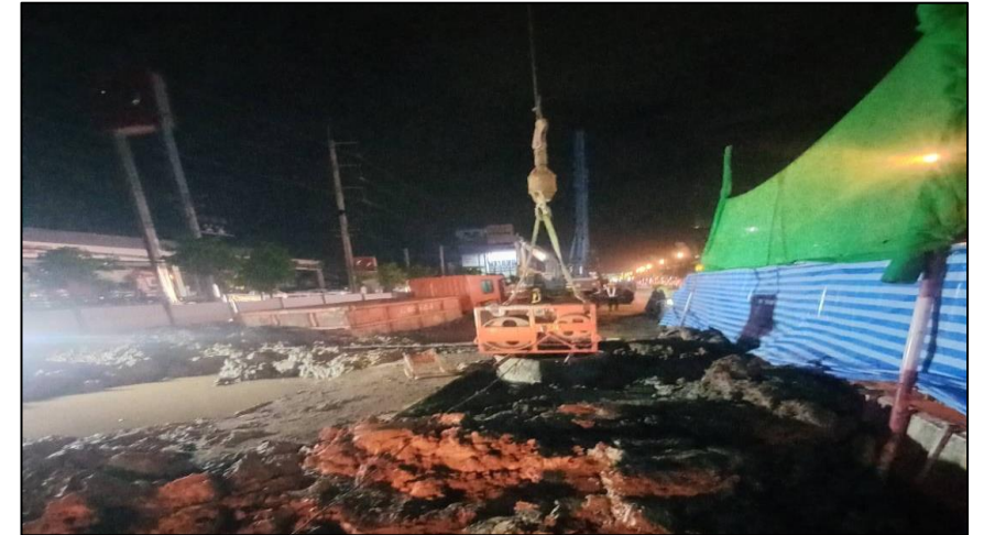
Drilling monitor Test Dia 1.00 m. RON2-01/2
