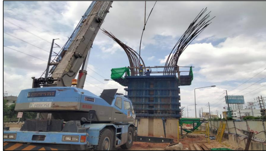
Install Steel Column Pier Type Y-1 Step 2 MLP05-09C
