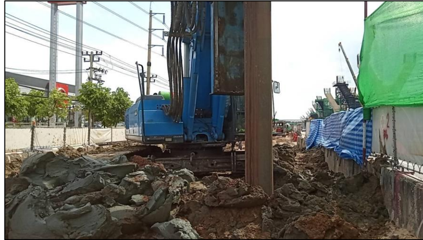
Grabbing Bored pile Dia 1.00 m. BP-1R/2
