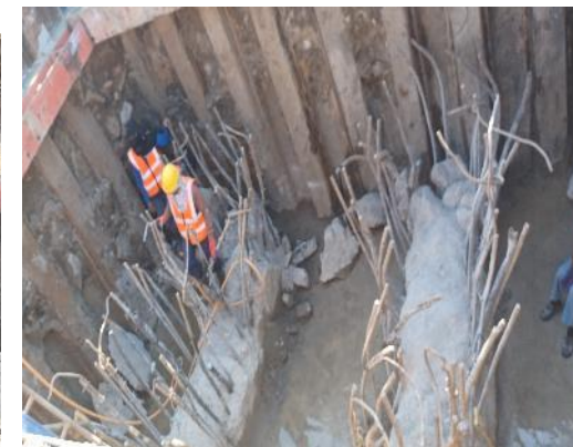
MLP01-21L Pile Cut Off
