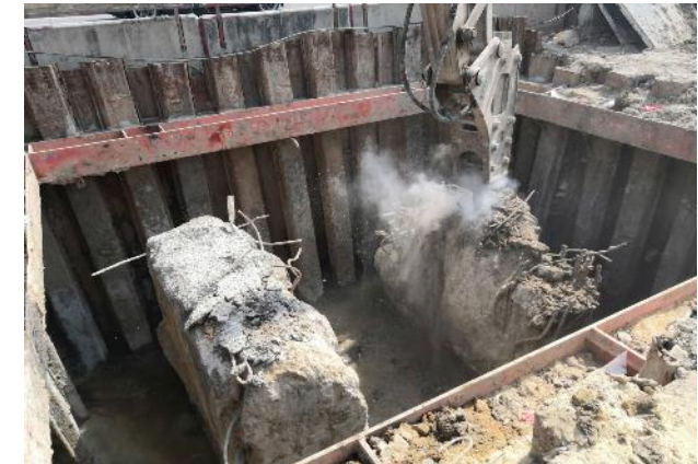
MLP01-16L Pile Cut Off
