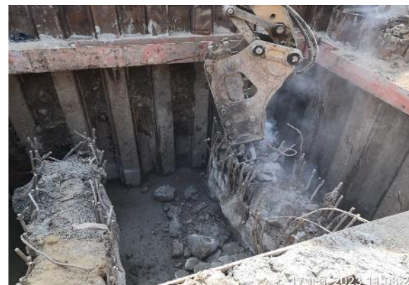
MLP01-21L Pile Cut Off
