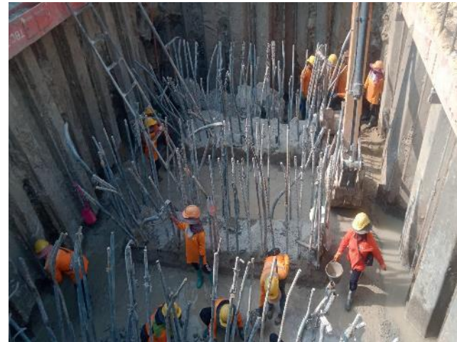
MLP01-15L Pile Cut Off
