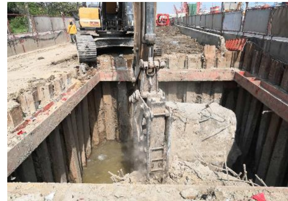
MLP01-16L Pile Cut Off
