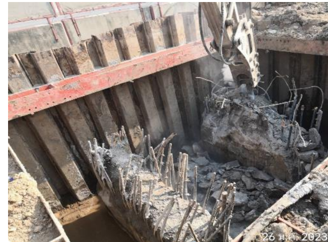
MLP01-17L Pile Cut Off
