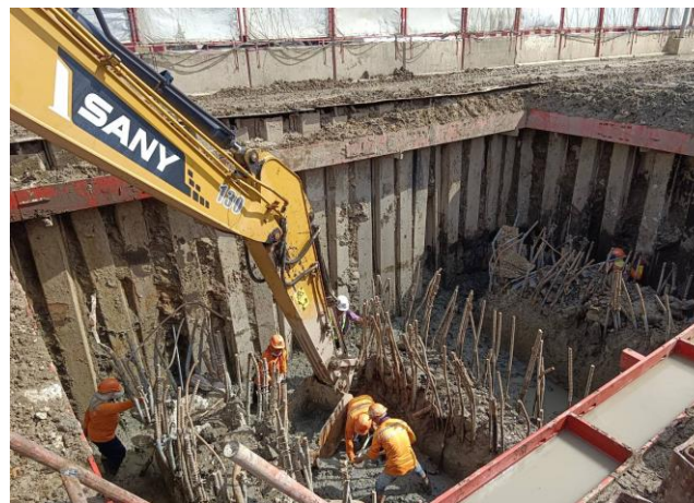
MLP01-22 Pile cut off
