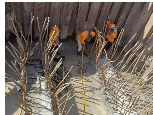
MLP01-21 Pile cut off
