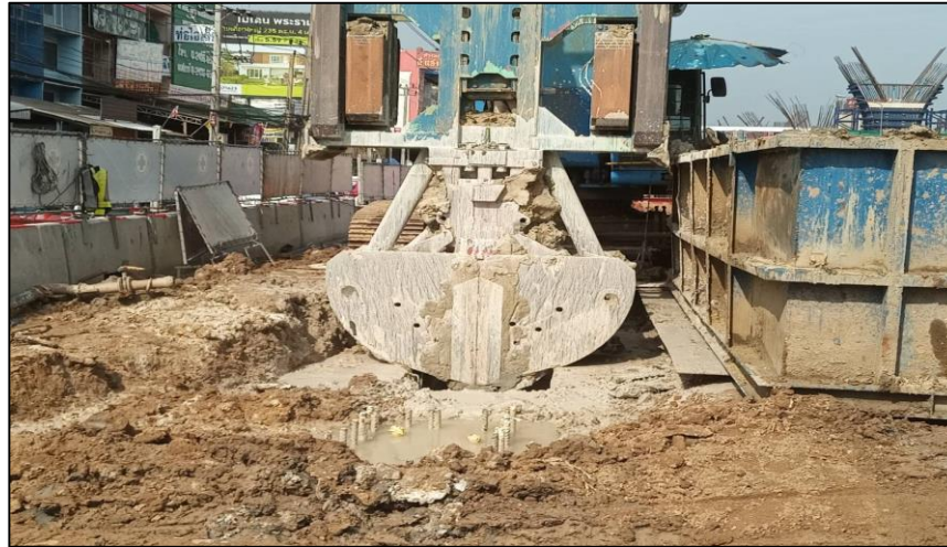
Grabbing Barrette pile 3.00x1.00 m. RON2-04/2
