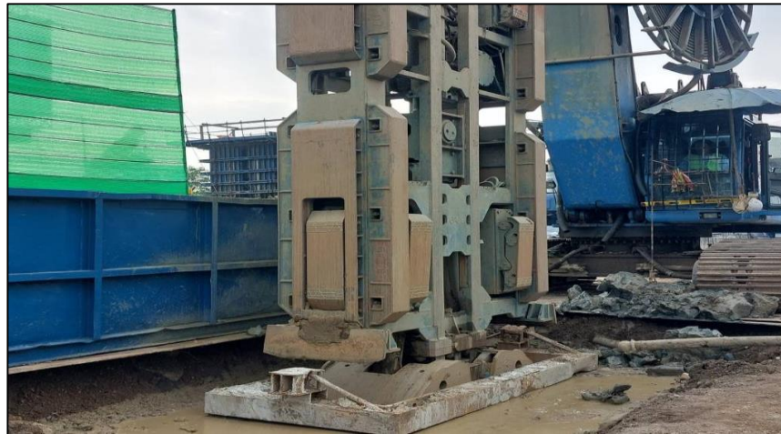
Grabbing Barrette pile 3.00x1.00 m. RON2-06/1
