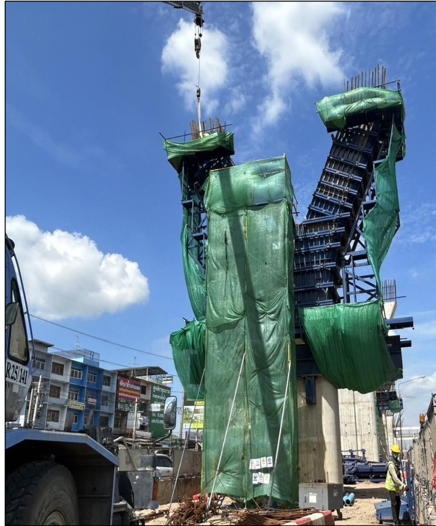
Install Steel Column Pier Type Y-1 Step Y MLP04-26C
