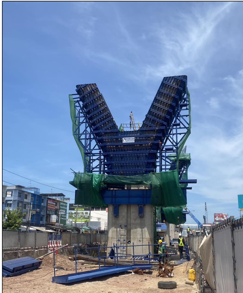
Install Steel Column Pier Type YT-1 Step Y MLP04-27C
