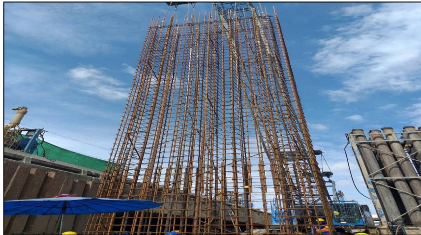
Install Rebar Barrette pile 3.80x1.00 m. MLP06-07C/1
