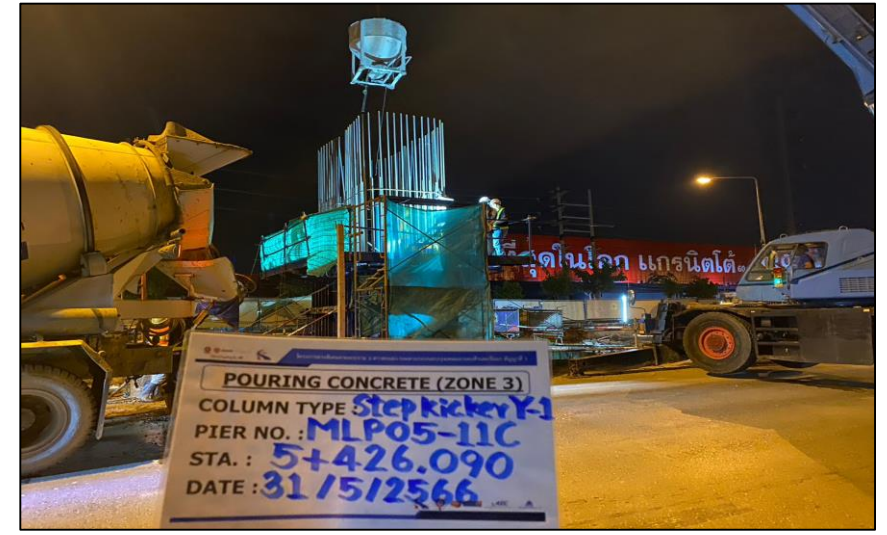
Pouring Concrete Column Pier Type Y-1 Step 1 MLP05-11C
