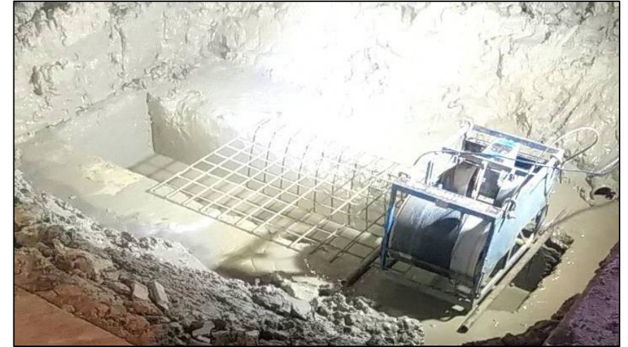
Drilling monitor Test MLP06-07C/1
