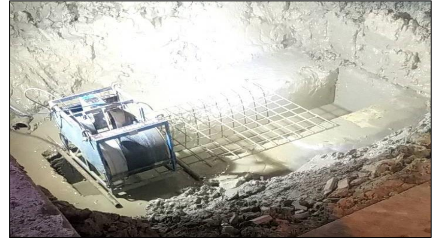
Drilling monitor Test MLP06-06C/3
