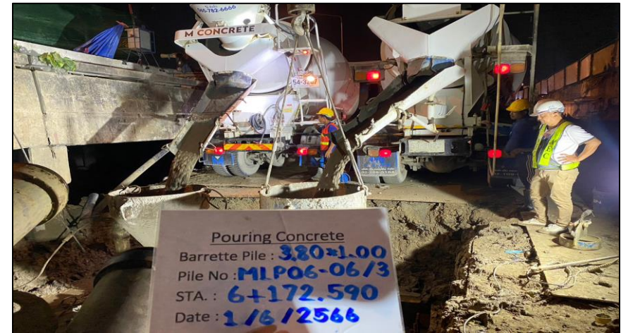
Pouring concrete Barrette pile MLP06-06C/3
