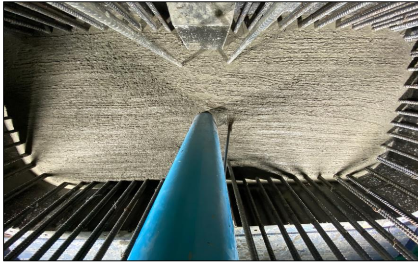
Pouring Concrete Column Pier Type Y-1 Step 1 MLP05-11C
