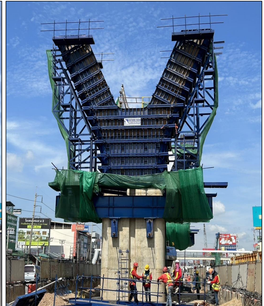
Install Steel Column Pier Type YT-1 Step Y MLP04-27C
