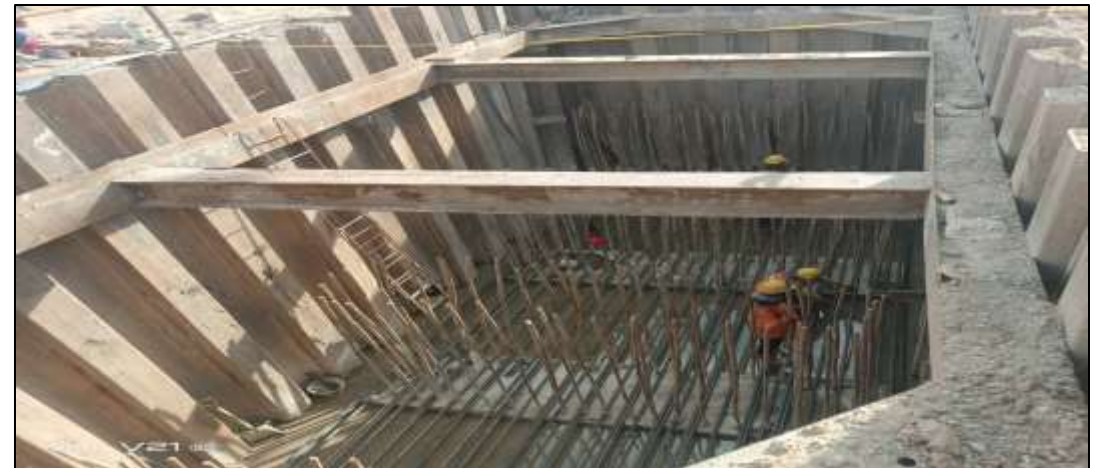
Pile cut off Footing 2F 3.00x1.00 m. No. MLP04-16C
