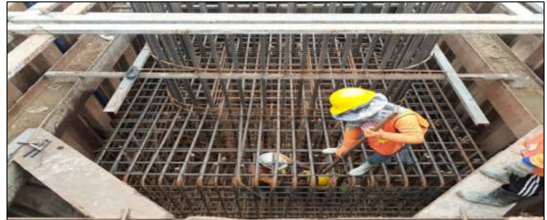
Installation Reinforcement Footing 2F 3.00x1.00 m. MLP04-18C
