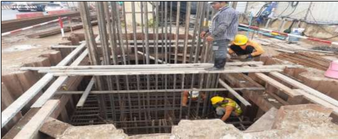
Installation Reinforcement Footing 2F 3.00x1.00 m. MLP04-18C
