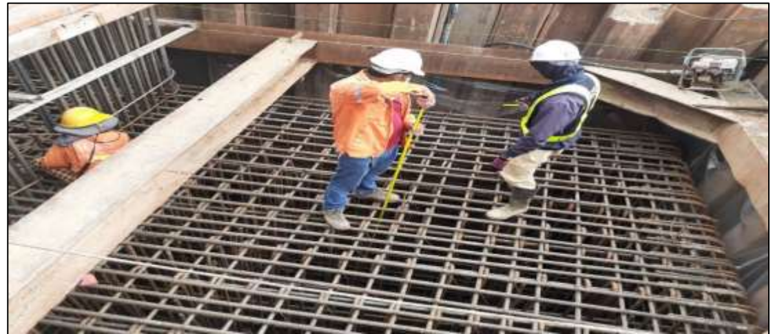
Installation Reinforcement Footing 4F 3.80x1.00 m. No. MLP04-15C
