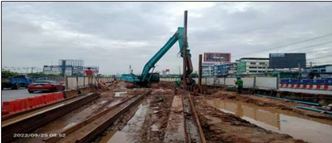
Excavation and Backfill for Structures included sheet pile MLP04-20C
