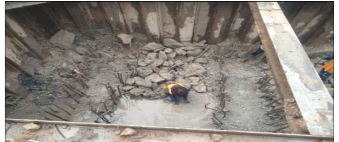
Excavation and Backfill for Structures included sheet pile MLP04-20C
