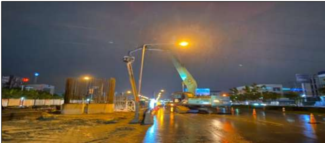
Remove sheet pile MLP05-06C
