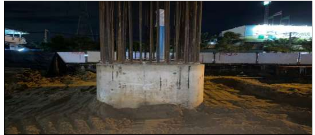
Backfill for Structures included sheet pile MLP05-06C
