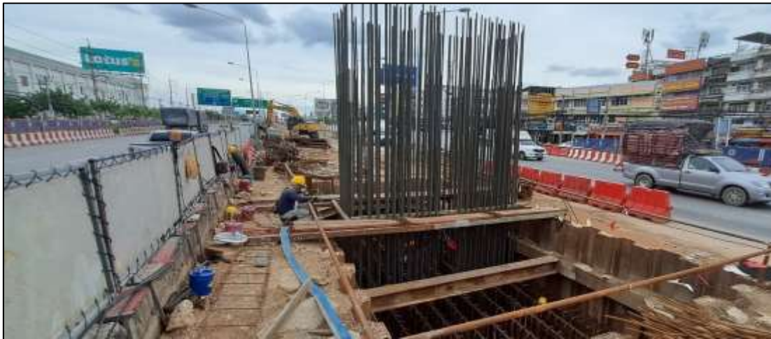
Installation Reinforcement Footing 4F 3.80x1.00 m. No. MLP04-15C
