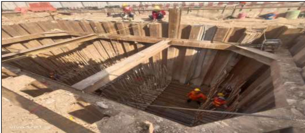
Pile cut off Footing 2F 3.00x1.00 m. No. MLP04-16C
